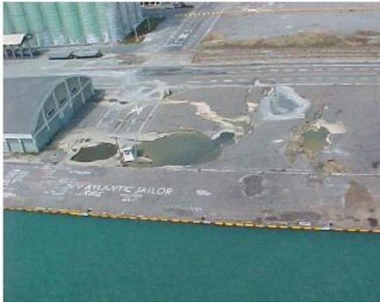
**Figure 1.5 :** Soil deformation behind quay wall at the port of Taichung during the 1999 Chi Chi earthquake
