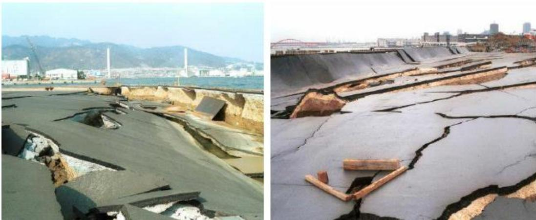
**Figure 1.2** : Substantial damages in the pavement, placed in the foot of quay walls during Kobe, Japan 1995 earthquake
