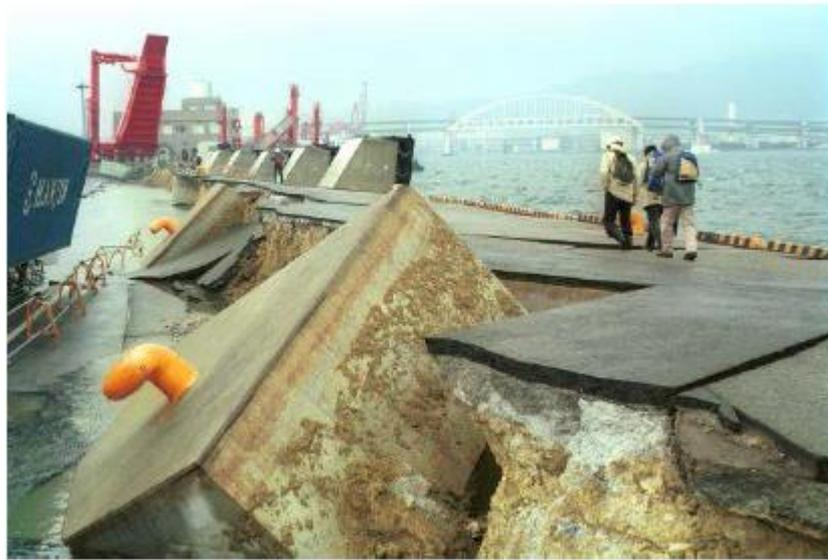
**Figure 1.4** : Overturn and great extent of quay wall's incline in Kobe 1995 earthquake
