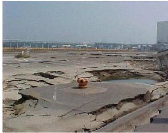
**Figure 1.6 :** Damages at the waterfront because of quay wall's displacement in 1999 Chi Chi earthquake
