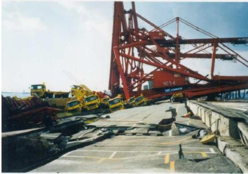
**Figure 2.21:** Damage to a quay wall at the Port of Kobe during the 1995 Hyogo-ken Nanbu Earthquake
