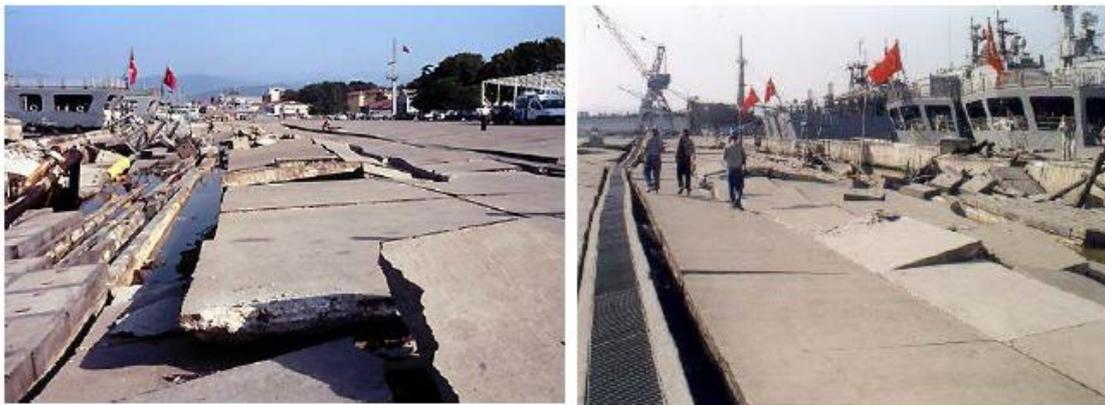
**Figure 1.4** : Damaged quay walls at Navy Seals' base of Gölcük in the 1999 Kocaeli earthquake in Turkey
