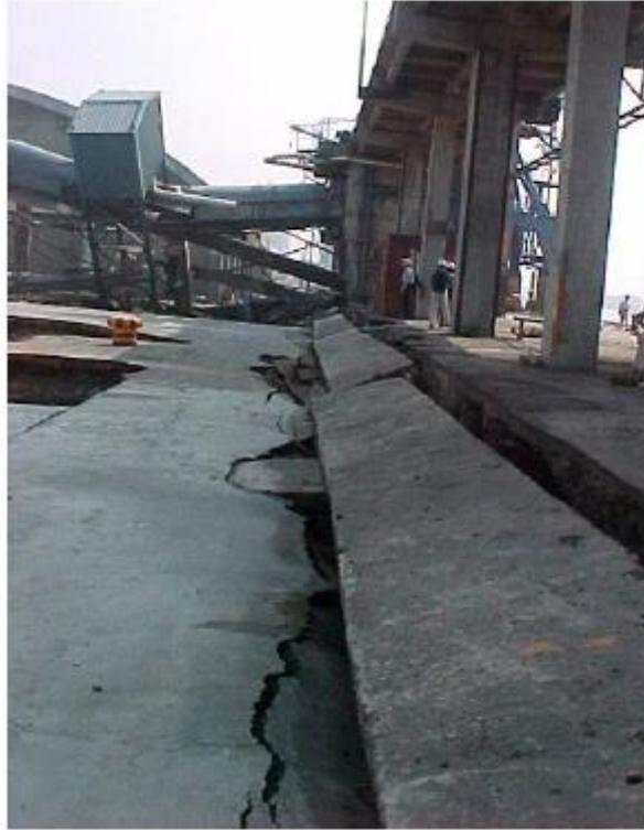
**Figure 1.5** : Settlement behind caisson-type quay wall in the port of Taichung, who suffered large displacement in 1999 Chi Chi earthquake
