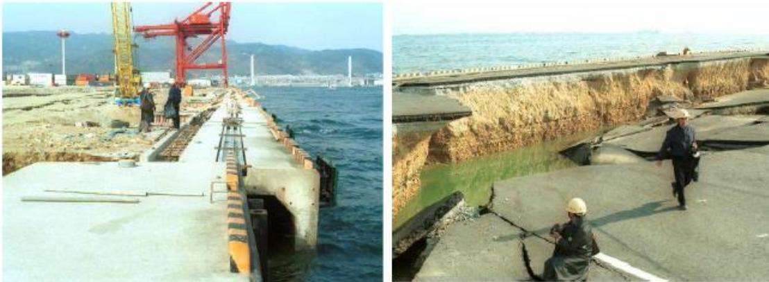
**Figure 1.1** : Quay walls displacement and incline to the sea at Kobe, Japan 1995 earthquake
