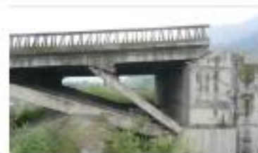
(f) shear damage of the ribs
