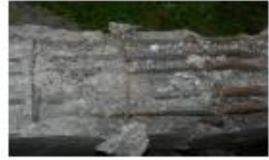
j) shear and slip damage (k) crack and inclines of the abutment(South) (l) stirrup hopping of the ribs
