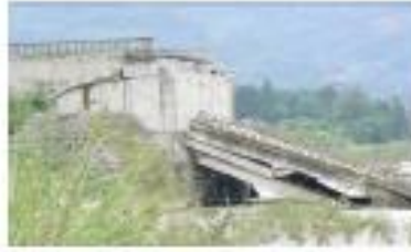
j) shear and slip damage (k) crack and inclines of the abutment(South) (l) stirrup hopping of the ribs
