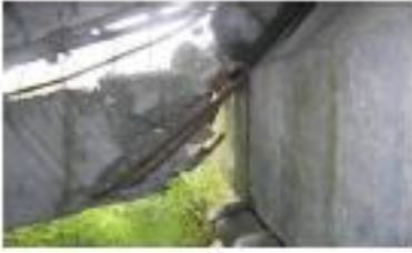
j) shear and slip damage (k) crack and inclines of the abutment(South) (l) stirrup hopping of the ribs
