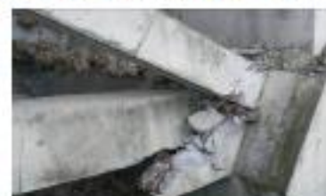
(f) shear damage of the ribs
