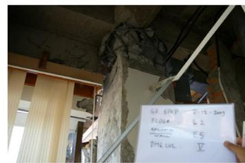
Photo 5. Damage degree III
