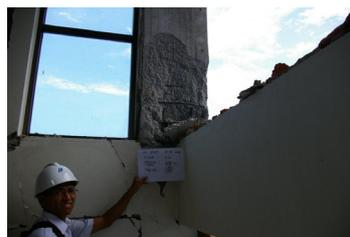
Photo 4. Damage degree IV
