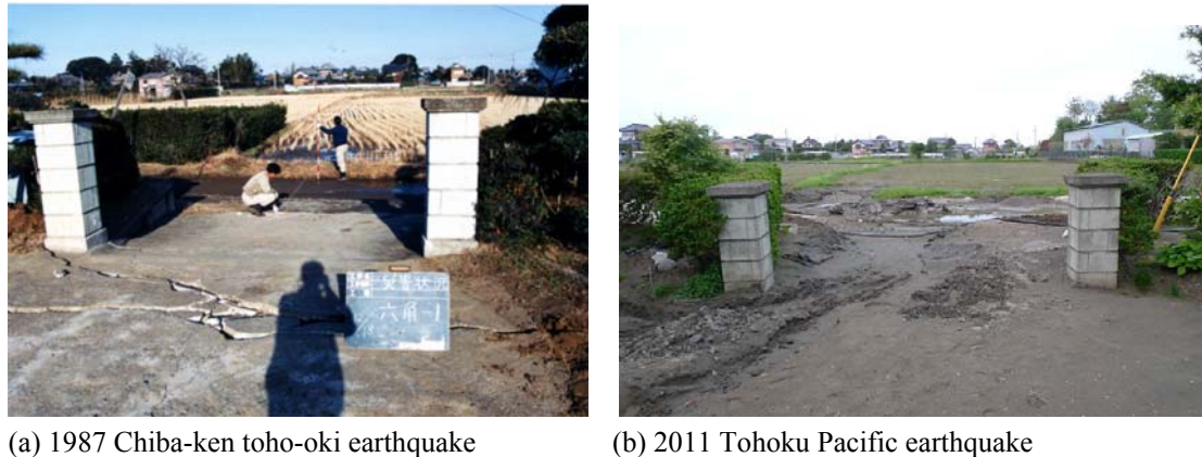
Figure 10 Liquefaction at same sites during the 1987 and 2011 earthquakes (Inashiki city, Ibaraki Prefecture)
