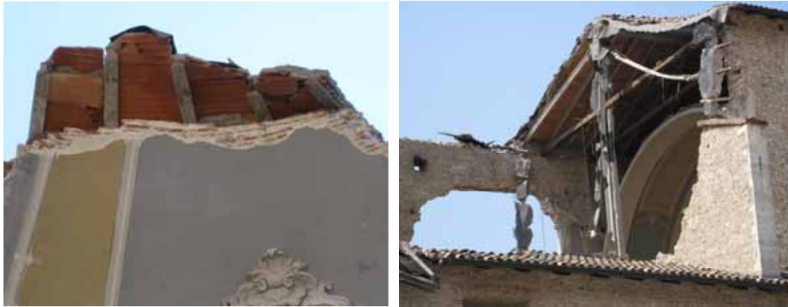
Figure 7. The modern roof made by r.c. precast elements and unreinforced concrete slab in Santa Maria Paganica church in L'Aquila: a) the small portion over the dome which did not collapse; b) trusses with pre-cast r.c. joists.
