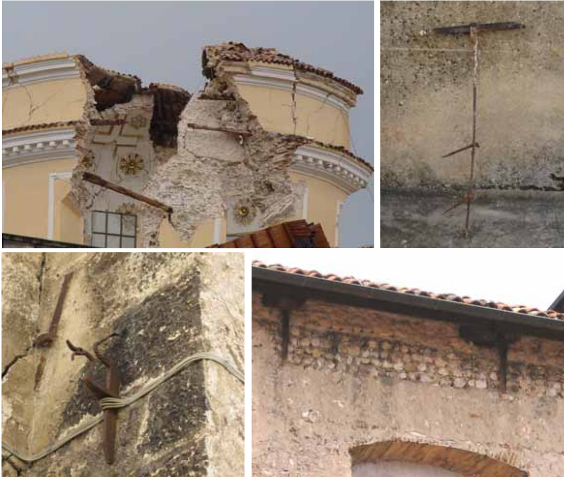
Figure 6. Some examples of “wooden ties” and connections: a) “wooden ties” at different levels of the dome of Santa Maria del Suffragio church in L’Aquila; b) the terminal connection elements, taken from the debris: the key and the steel plate (with two nails); c) the external key; d) and external wooden key for the connection of the trusses in Santa Maria del Carmine church in L’Aquila.
