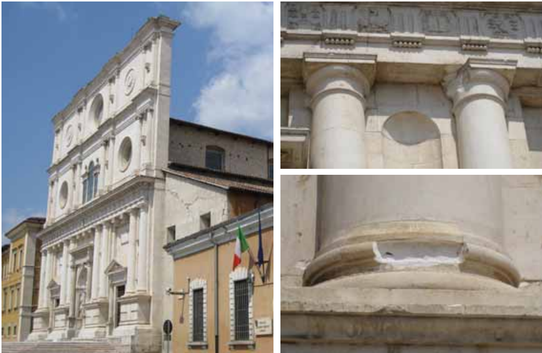
Figure 9. S. Bernardino basilica in L'Aquila: a) the façade; b-c) details of some local crushing of marble elements due to out-of-plane overturning mechanism.
