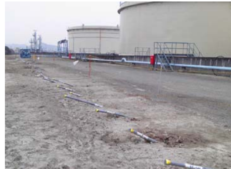
(b) Installed grouting pipes
