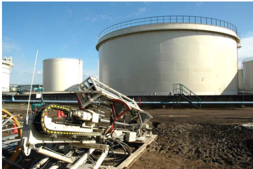
(a) Directional drilling towards the ground beneath the tank
