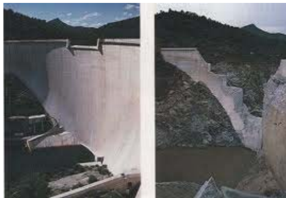
Figure 1. Malpasset dam (before and after the collapse, MA 1960).
