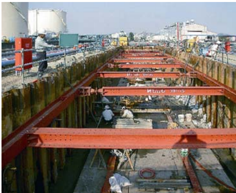
Figure 3. Conventional horizontal grouting from a vertical shaft
