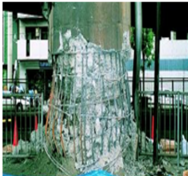
Cover concrete suffered and outer longitudinal bars buckled.
