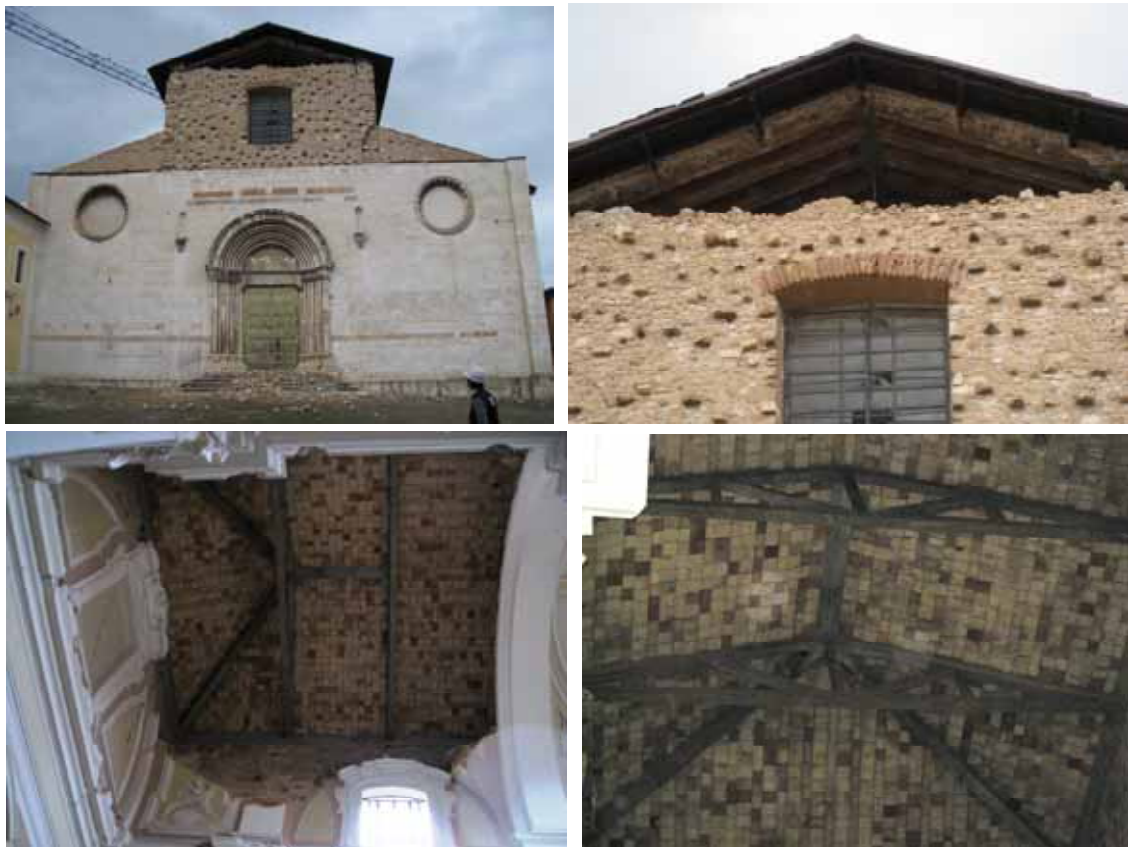
Figure 11. San Domenico church in L'Aquila: a) the facade; b) the collapsed gable of the facade; c-d) collapse of the transept vault due to substitution of the roof, made by r.c. trusses.
