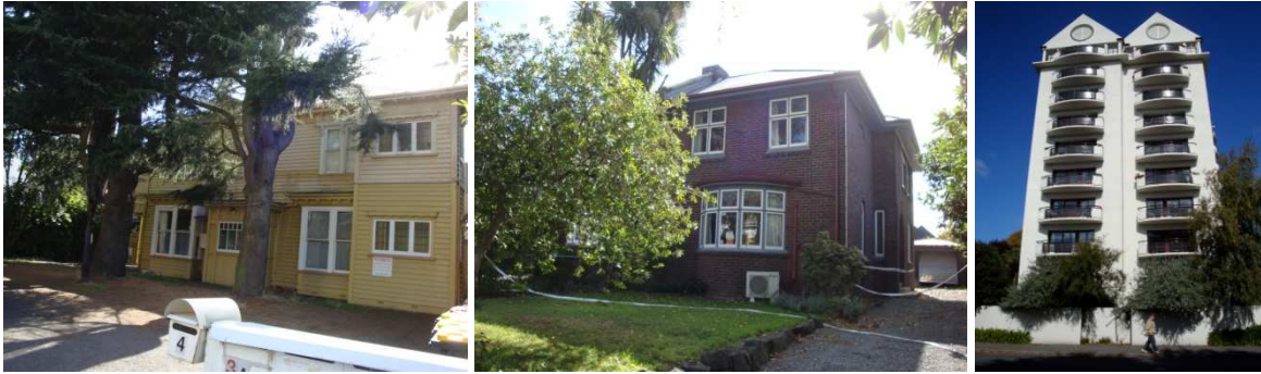
Figure 7. Characteristic timber (left), masonry (middle) and modern RC (right) structures outside of CBD.
