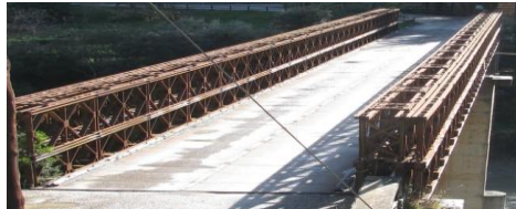
Photo 6. The triple-double Bania bridge
