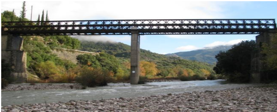
Photo 2. The Bania bridge in its present form
