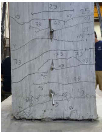
Figure 4. SMA/ECC column plastic hinge damage after 12% drift cycles
