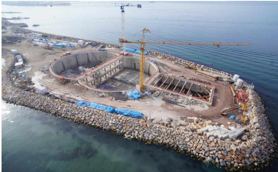
Figure 17. South anchor block after completion of excavation and initial concreting at the base
