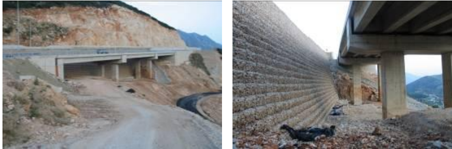
Photos 1,2. The G2/Kristallopigi bridge on Egnatia Motorway.
