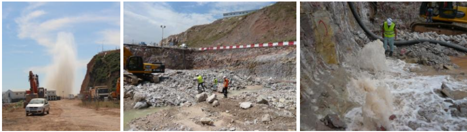
Figure 10. Excavation for North anchor block, (a) Blasting from a safe distance; (b) Debris after blasting; (c) Major water ingress in north wall after blasting
