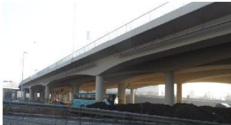
Photo 4. NAR – Viaducts over J. Gagarina street
