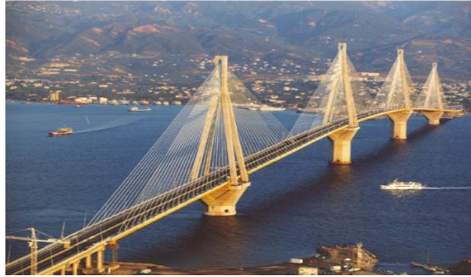
Photo 1. Rion - Antirion bridge
