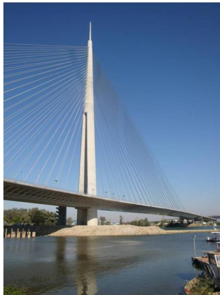
Photo 2. Ada Bridge (by day)
