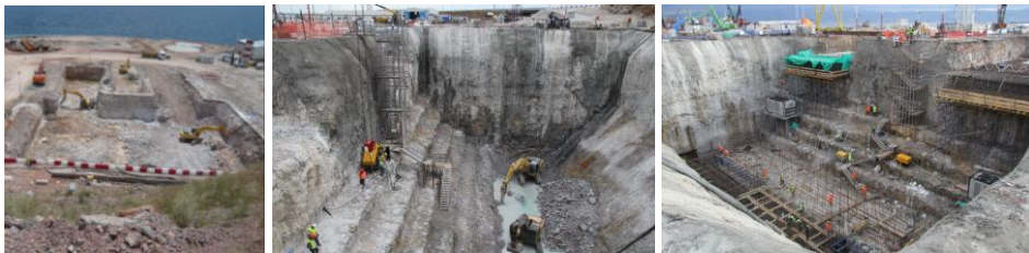
Figure 11. North anchor block excavation and casting of front pads and base
