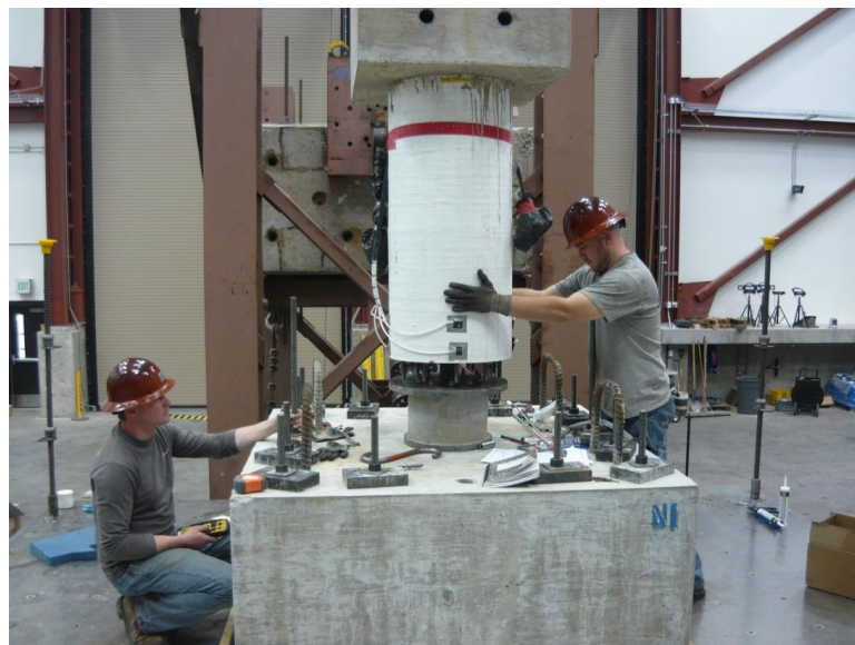
(c) Installing precast concrete-filled FRP tube segment
