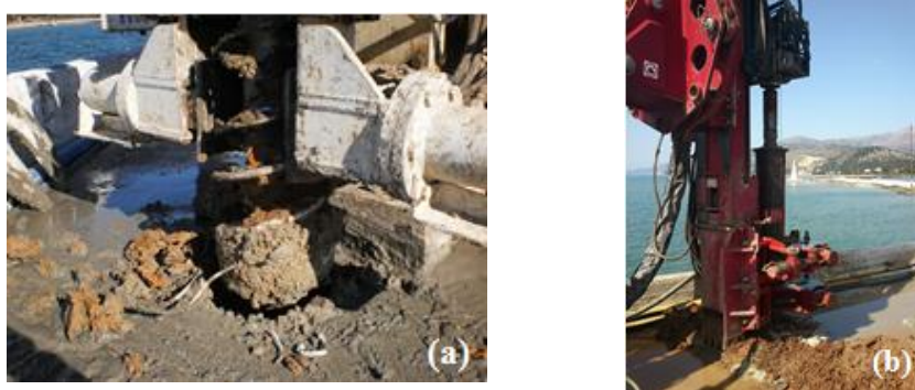
Figure 5. (a) Filling material of the bridge revealed during restoration works (b) Steel tubes embedded consecutively to restrain debris fall inside the borehole during drilling
