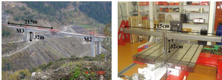
Figure 1. Metsovo Bridge segments during the construction stage (left) and its equivalent scaled structure tested at the laboratory (right).
