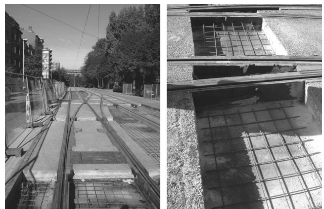
Fig. 3. Continuous rail support system (developed by Kihn-Cogifer) during construction
