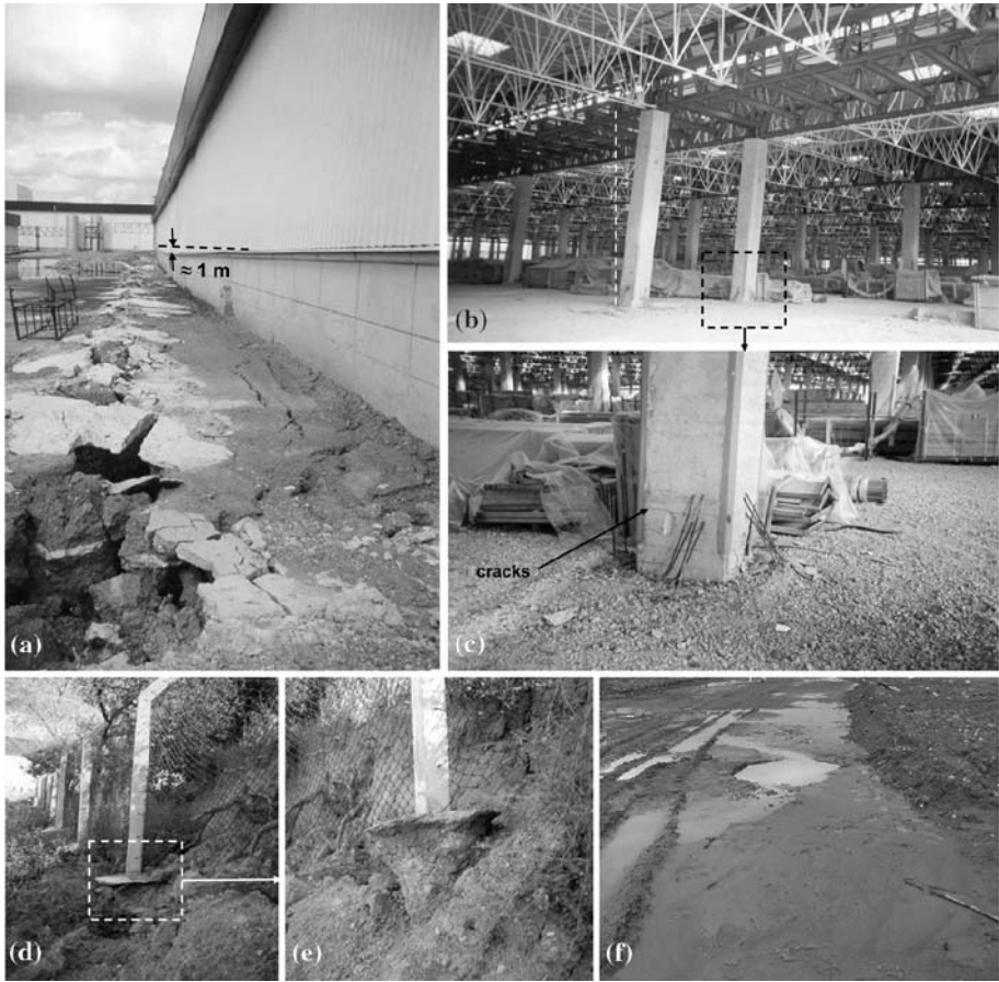
Fig. 3 Ford factory: (a) differential settlement of about 1 m, (b) tilting of concrete columns, (c) cracking at the base of the columns, (d) fault rupture right through the fence, (e) fence footing pulled out, (f) traces of liquefaction north of the building
