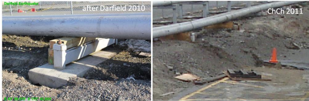
Figure 5.27. Comparison of the fuel pipe line deformation (site W3 in the map of Figure 5.6) between Darfield and Christchurch earthquakes. After Darfield earthquake, temporary wooden support was used to accommodate settlement under fuel line (Cubrinovsky et al., 2010). After Christchurch earthquake, the supports are still there and they have settled together with the fuel line.
