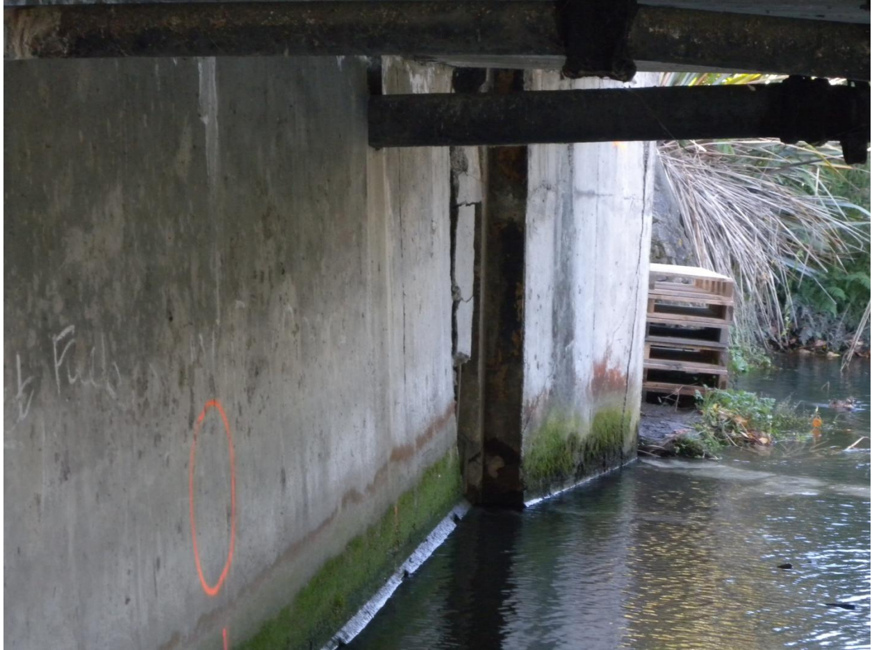
Figure 5.17. Northern abutment of Gayhurst Bridge (B4 on map of Figure 5.1). Rotation and differential riverward displacement (in the order of 70 cm and more) of the eastern wingwall relative to the abutment caused concrete spalling and cracking at the joint of the abutment with the wingwall.
