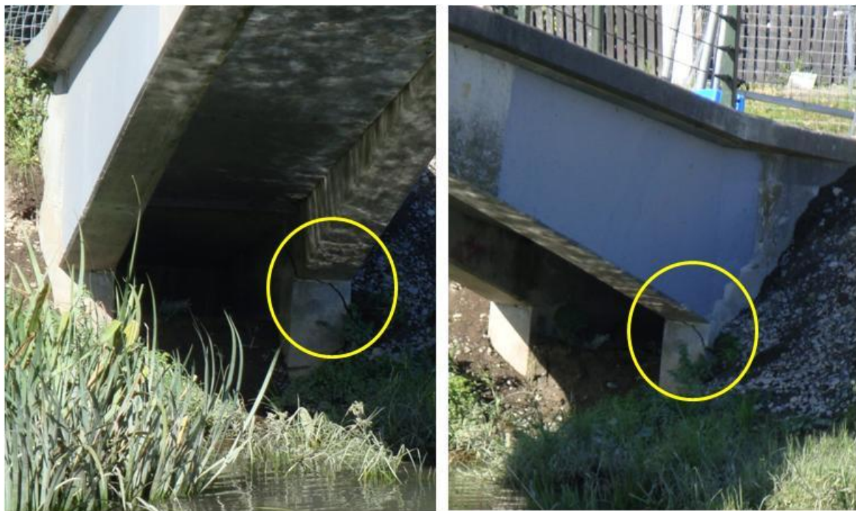
Figure 5.22. Snell Footbridge (B5 on map of Figure 5.1) after Christchurch earthquake. Cracks in the abutments.
