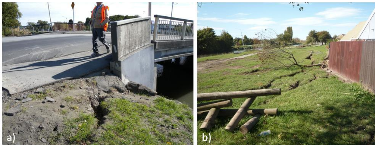
Figure 5.27. a) Back rotation of southern abutment of Avondale Bridge (B6 on map of Figure 5.1), cracks in the backfill, b) Large lateral spreading cracks in the south coast parallel to the river extending in a great distance at both sides of the southern abutment.
