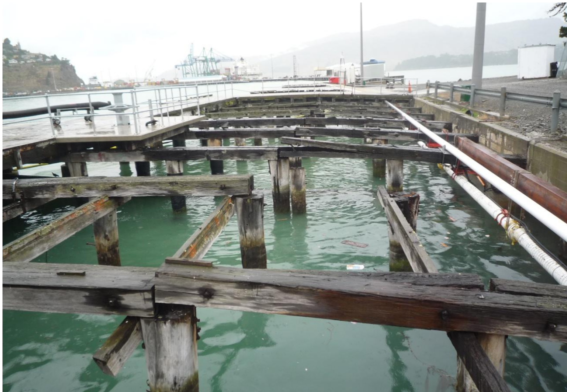
Figure 5.20. Settlement of the backfill caused detachment of the wooden beams from the pile heads (site W3 in the map of Figure 5.6).
