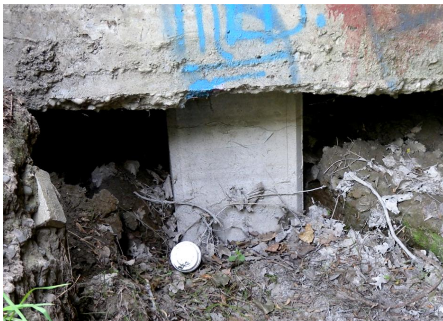
Figure 5.6. Fitzgerald Bridge (B1 on map of Figure 5.1). Rotation of northern abutment has caused tension cracks at the pile-tops.
