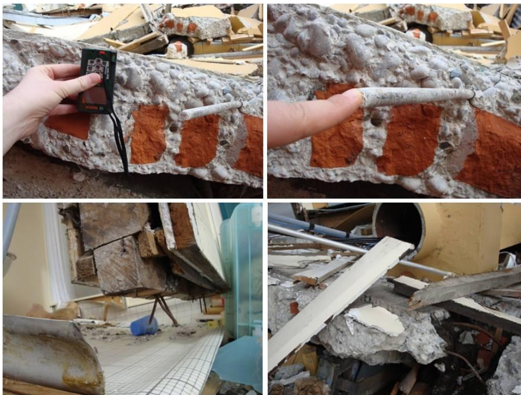
Figure 3. 8. The heavy external wall and the slab detail of the collapsed Stonehurst Hostel.
