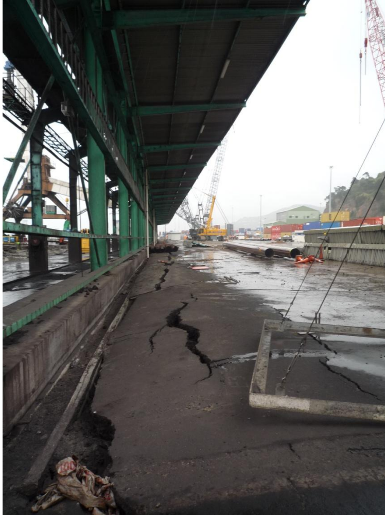
Figure 5.18. Large uniform settlement under the heavy load of the structure. Cracks in the asphalt due to heaving of the ground at right side of the steel structure (site W2 in the map of Figure 5.6)
