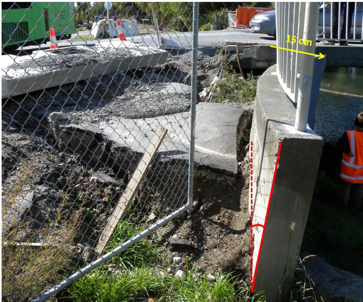
Figure 5.18. Northern abutment of Gayhurst Bridge (B4 on map of Figure 5.1). Rotation and displacement of the western wingwall not only riverwards but also away from the abutment (15 cm approximately at the top) perpendicular to the deck.
