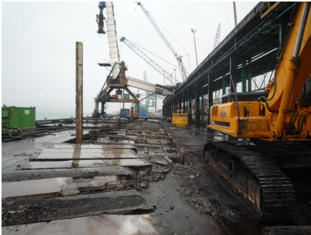
Figure 5.19. Detachment of the slabs of the platform due to differential settlement (site W2 in the map of Figure 5.6). Now the slabs have been removed from their initial place.
