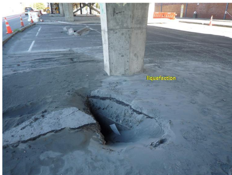
Figure 5.53. Sand-boils indicating liquefaction.
