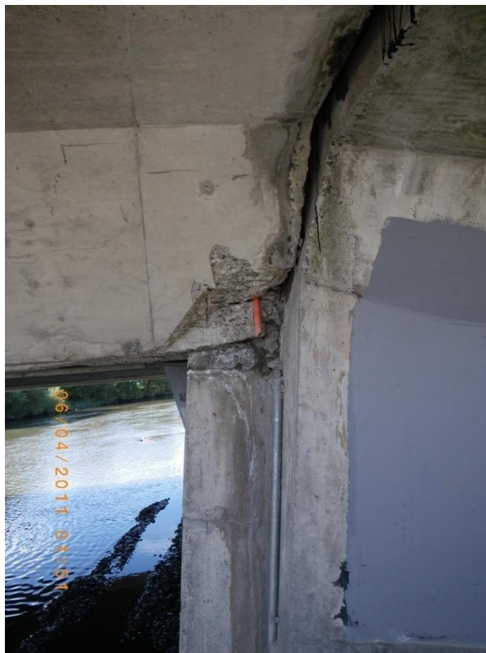
Figure 5.26. Southern abutment of Avondale Bridge (B6 on map of Figure 5.1) after Christchurch earthquake. Concrete spalling and gap opening at the joint of the deck with the abutment.
