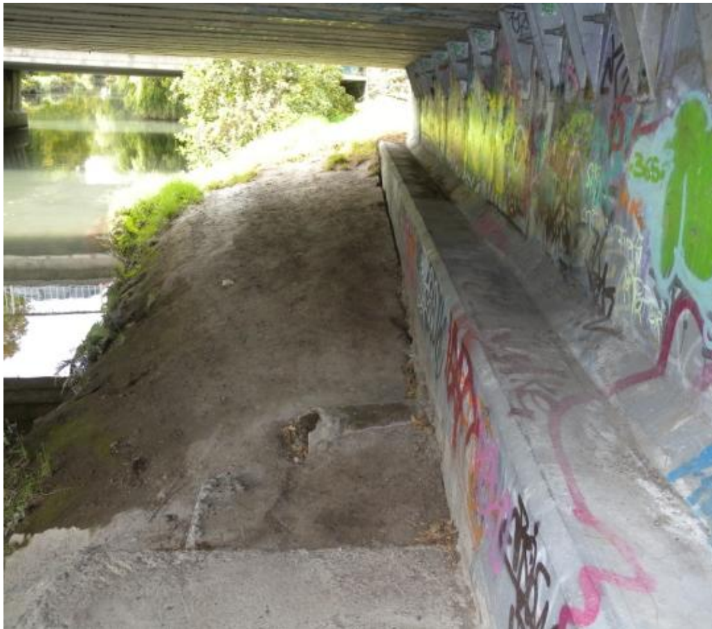
Figure 5.2. Fitzgerald Bridge (B1 on map of Figure 5.1). Performance of southern abutment after ChCh earthquake. No signs of lateral ground deformation occurred at the southern abutments of the twin bridges. The soil is still attached to the abutment.
