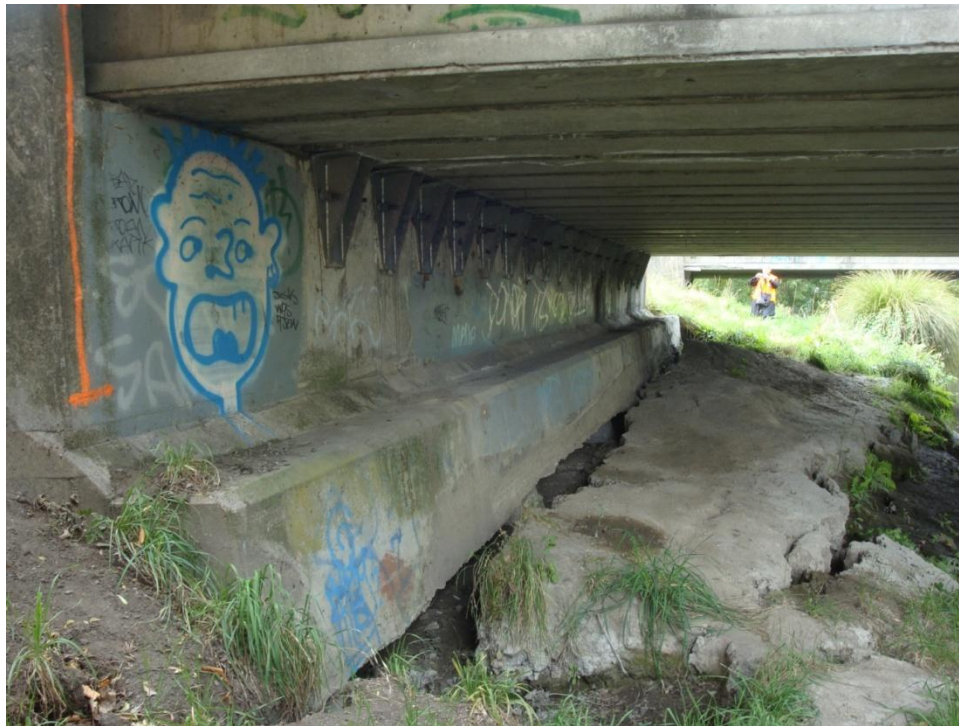
Figure 5.4. Fitzgerald Bridge (B1 on map of Figure 5.1). Performance of northern abutment after ChCh earthquake. Lateral spreading of the ground has exposed the pile heads.
