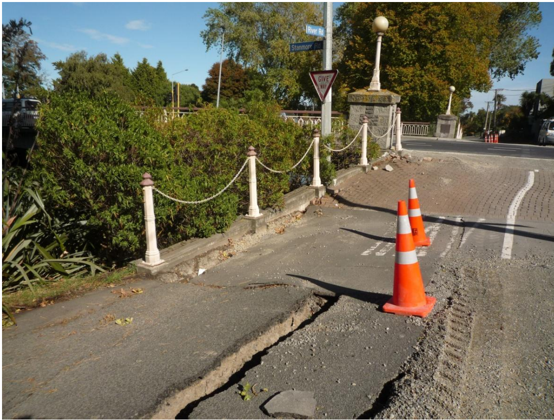
Figure 5.11. Stanmore Bridge (B2 on map of Figure 5.1). Rotation of the abutment around the deck. The street lighting column next to the abutment has rotated riverwards, following the lateral deformation of the ground, while the light column seated on the abutment indicates that the abutment has back rotated due to the deck constraint. Slump of the approach fill is not visible because at the time of our visit, the cracked asphalt between the two abutments had been replaced by new. However the large cracks in the road parallel to Avon river (in the order of 40 cm) due to lateral spreading were still there.
