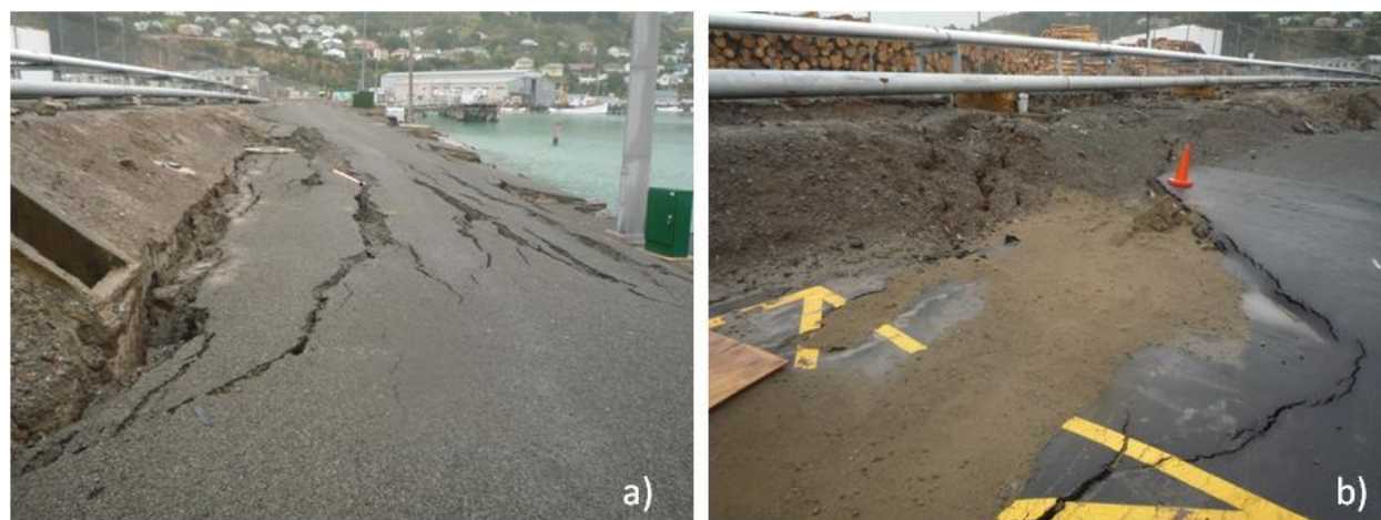
Figure 5.25. a) Cracks in the inclined asphalt due to lateral spreading, b) Ejected sand appeared on the surface indicating that liquefaction has occurred (site W3 in the map of Figure 5.6).
