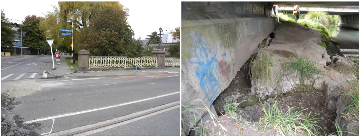
Figure 3. 2. Bridge at Oxford Terrace (left) and rotated abutment of Fitzgerald bridge (right).
