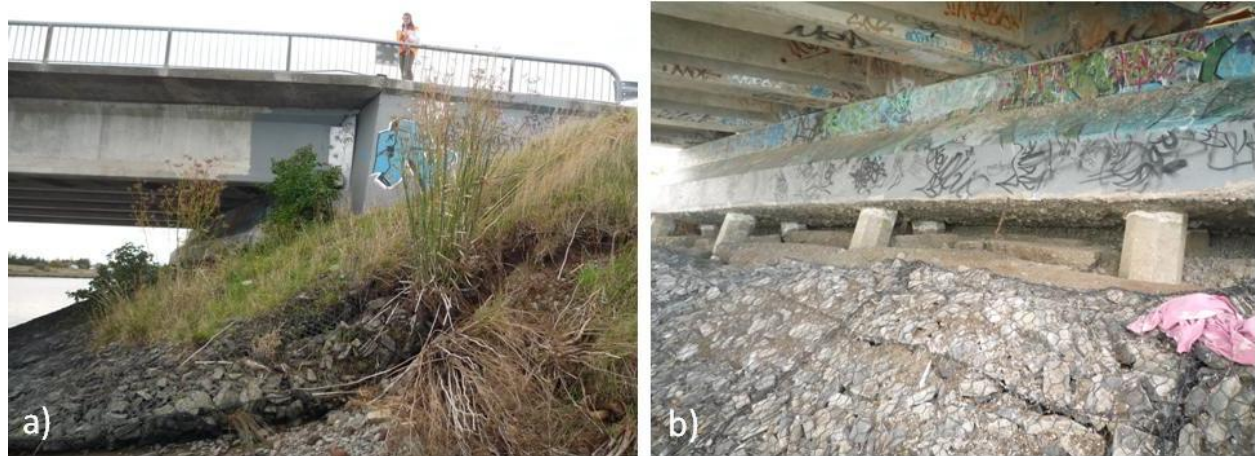
Figure 5.36. Eastern abutment of South Bridge Road Bridge (B8 on map of Figure 5.1) after Christchurch earthquake. a) Back rotation of the abutment around the deck and slump of the approach fill, b) the soil underneath the abutments has moved riverwards exposing both rows of piles.
