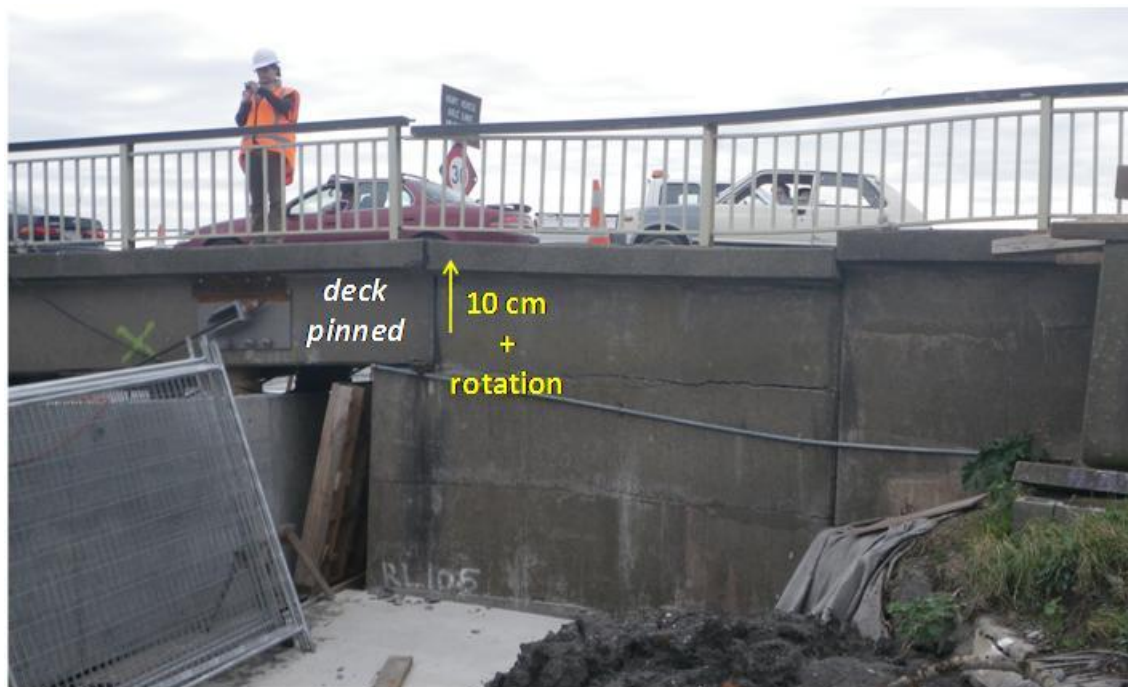
Figure 5.45. East abutment of Ferrymead Bridge after Christchurch earthquake (B8 on map of Figure 5.1). The front section of the abutment has back rotated and moved upwards by 10 cm. The rear section of the abutment has been displaced in a similar trend.
