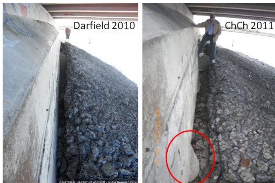
Figure 5.41 Western abutment of South Bridge Road Bridge (B8 on map of Figure 5.1). Differences between Darfield and Christchurch shaking events. After Christchurch earthquake,
