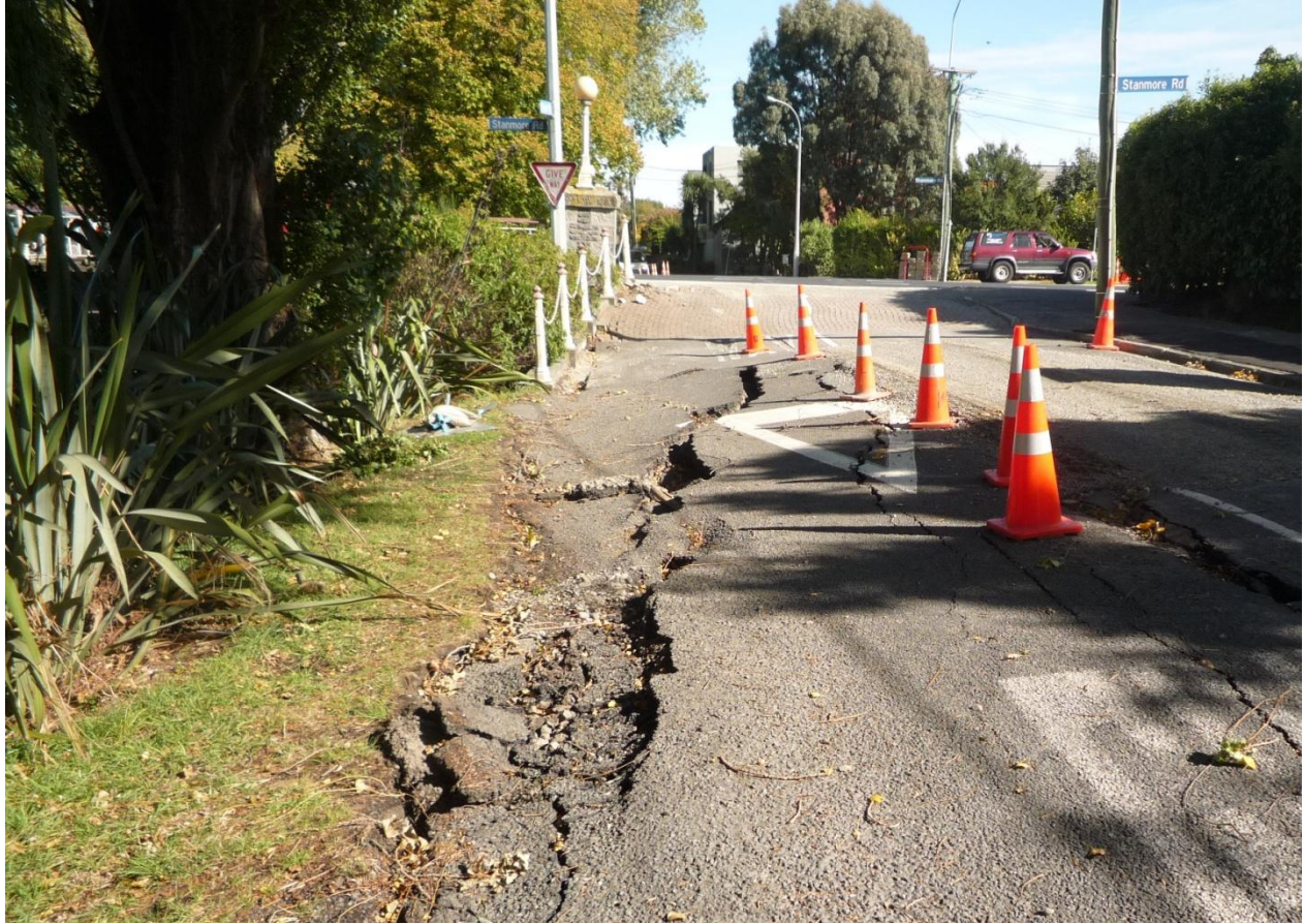
Figure 5.12. Stanmore Bridge (B2 on map of Figure 5.1). Large cracks in the asphalt due to significant lateral spreading in the free field (away from the bridge). The cracks tend to decrease towards the bridge, as the axial stiffness of the deck combined with the bending stiffness of piles limits the lateral ground deformation.
