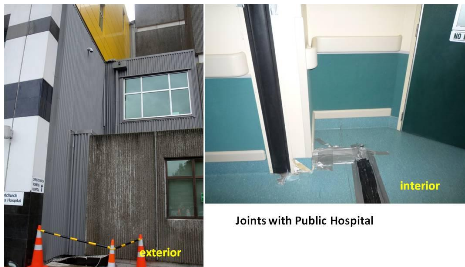
Figure 3. 46. Non-structural detailing in Women's Hospital to allow differential displacements due to the isolators.
