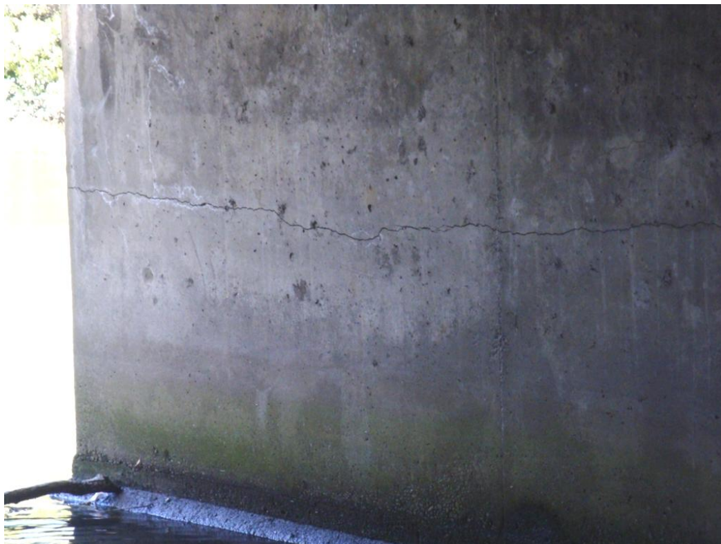
Figure 5.16. Gayhurst Bridge (B4 on map of Figure 5.1) The pier wall close to the northern abutment developed horizontal tension cracks, about 1 m below the deck due to intense shaking and lateral spreading.
