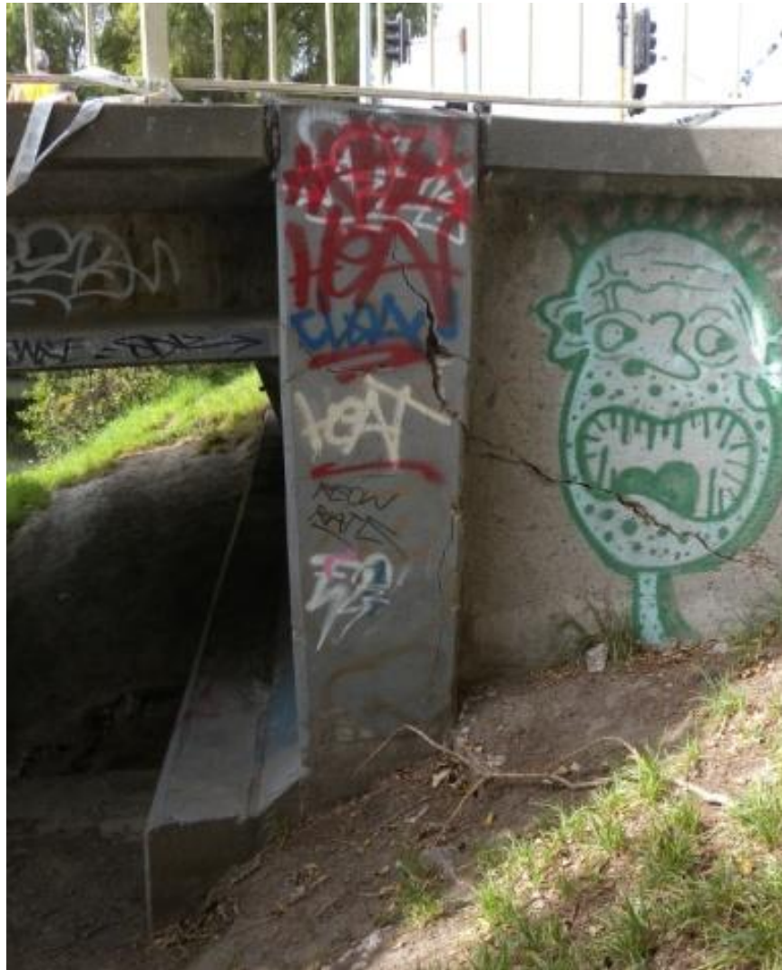
Figure 5.3. Fitzgerald Bridge (B1 on map of Figure 5.1). Performance of southern abutment after ChCh earthquake. No lateral ground deformation occurred at the southern abutments of the twin bridges. Thus, there was no rotation of the abutment. However, the southern abutment suffered moderate cracks due to seismic and inertial load.
