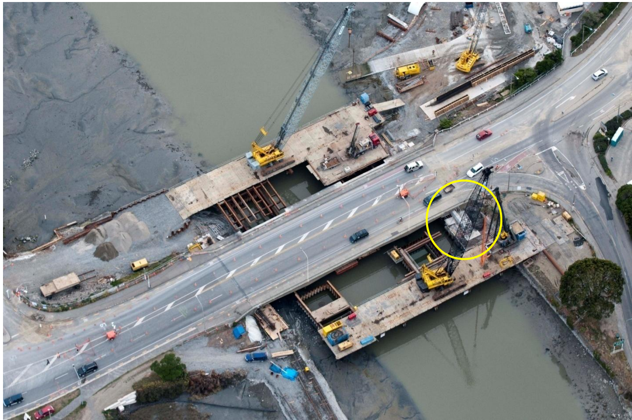
Figure 5.43. Ferrymead Bridge (B8 on map of Figure 5.1). Construction site in the process of strengthening and widening of the bridge. Photo taken after Christchurch earthquake. The new east abutment, in the yellow circle, was built one month before the shaking event.
