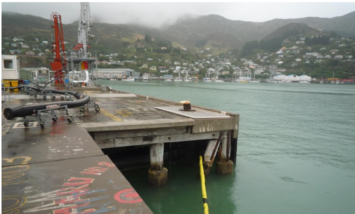
Figure 5.22. Another typical pile configuration (site W3 in the map of Figure 5.6). The concrete piles performed quite well.
