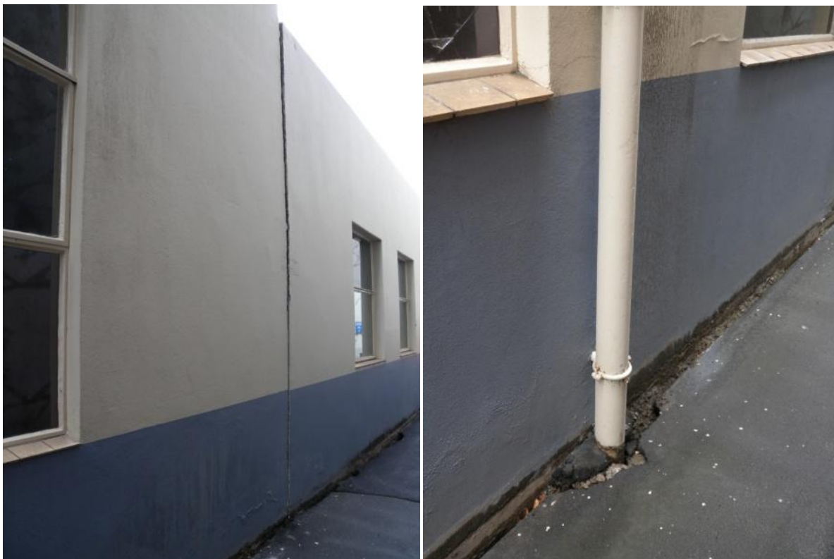
Figure 2.15. Gap opening between the front and rear section of CHHC seismic station building (left). Crack between the building and the asphalt due to ejected sand (right).
