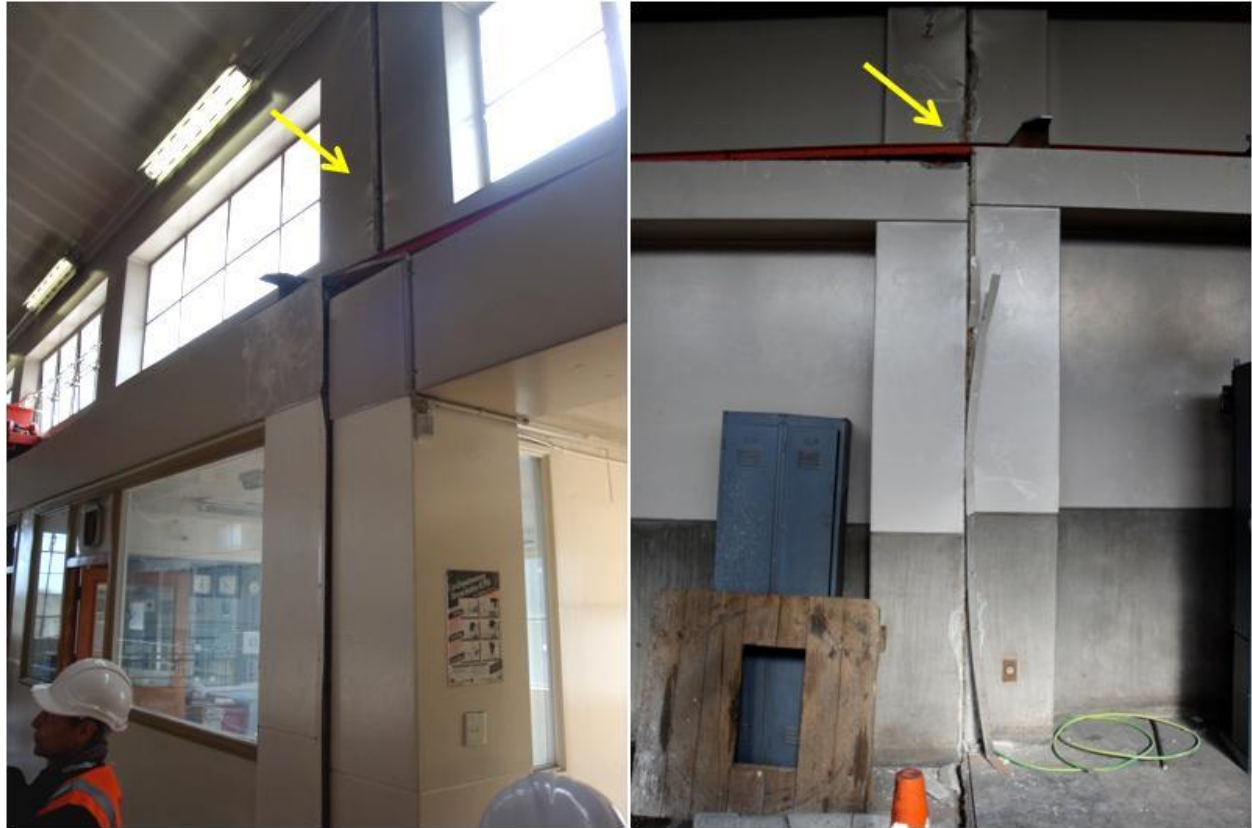
Figure 2.43. Interior of the Pumping Station next to the garage. Differential movement at the joint of one section of the building with the other.
