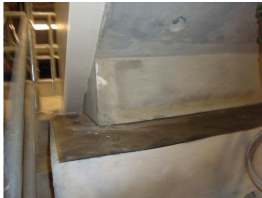
Figure 3. 44. Detail of the staircase that connects the isolated floor with the rest of the building (the sitting part of the stairs is allowed to slide freely)
