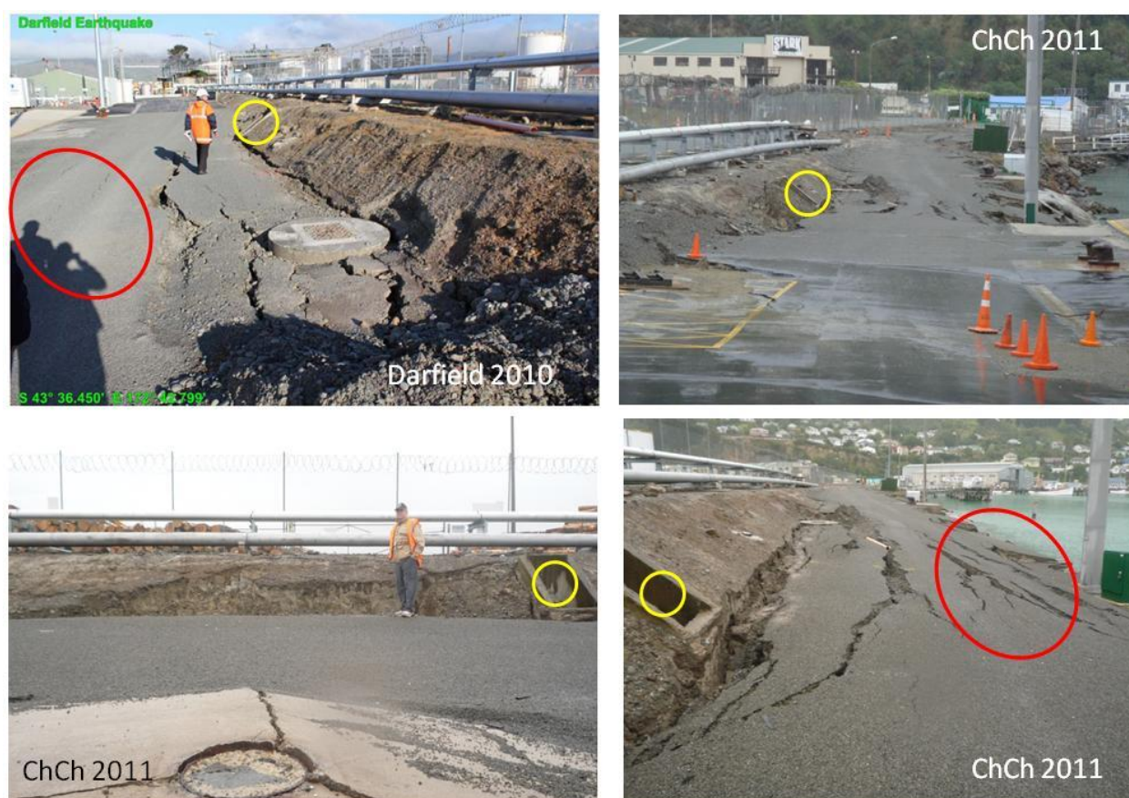
Figure 5.26. Comparison of the damage of site W3 in the map of Figure 5.6 between Darfield and Christchurch earthquakes. The yellow and red circles are the common point of references in all photos. Photo from Darfield earthquake can be found in Cubrinovsky et al. (2010).
