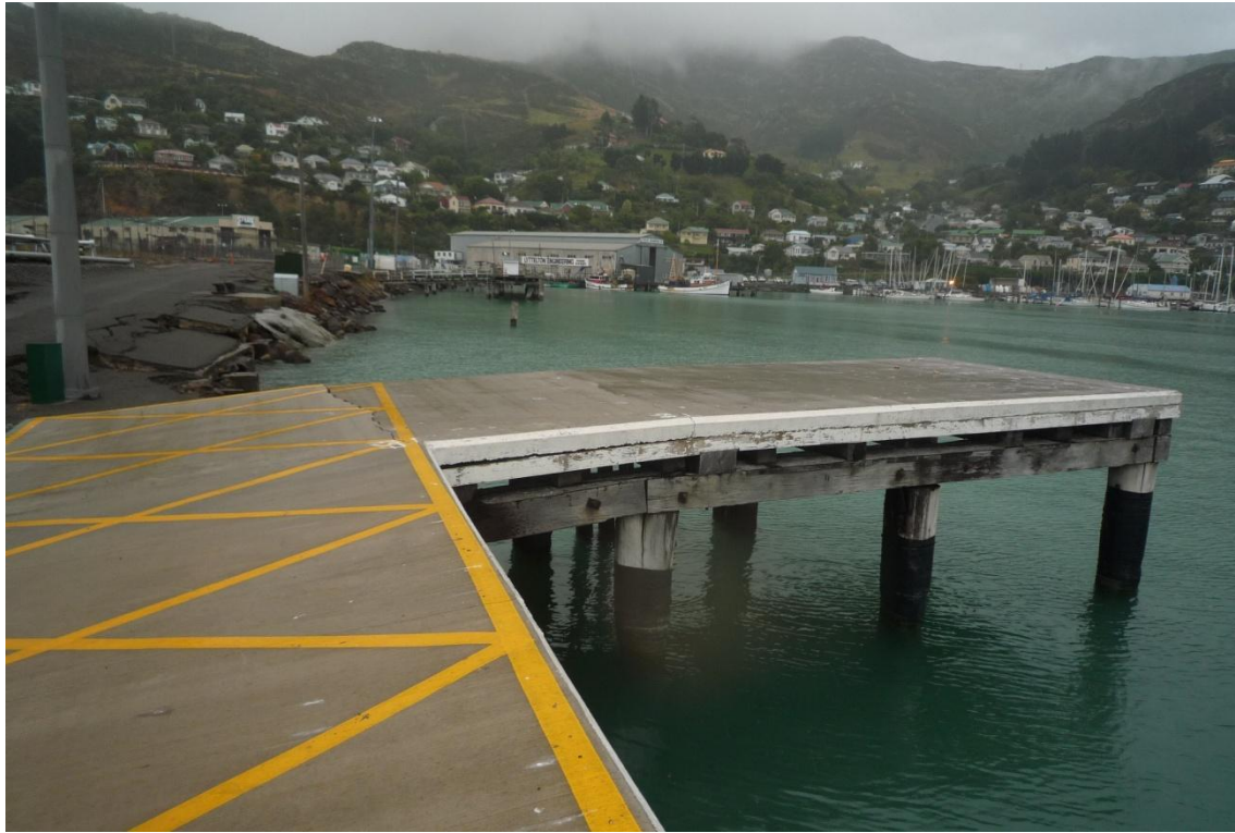
Figure 5.21. One typical pile configuration (site W3 in the map of Figure 5.6). The timber piles have cracked at the top.
