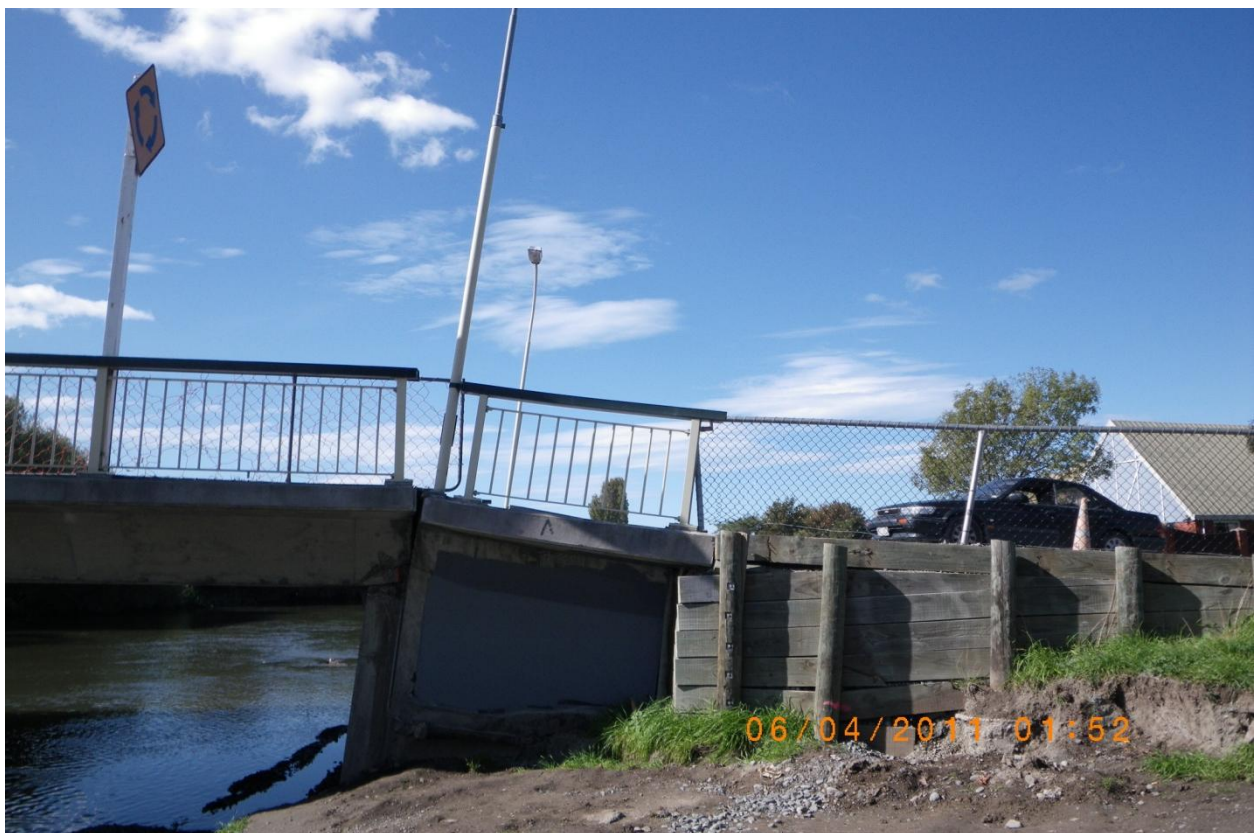
Figure 5.25. Southern abutment of Avondale Bridge (B6 on map of Figure 5.1) after Christchurch earthquake. Back rotation (8 degrees) and subsidence of the backfill.
