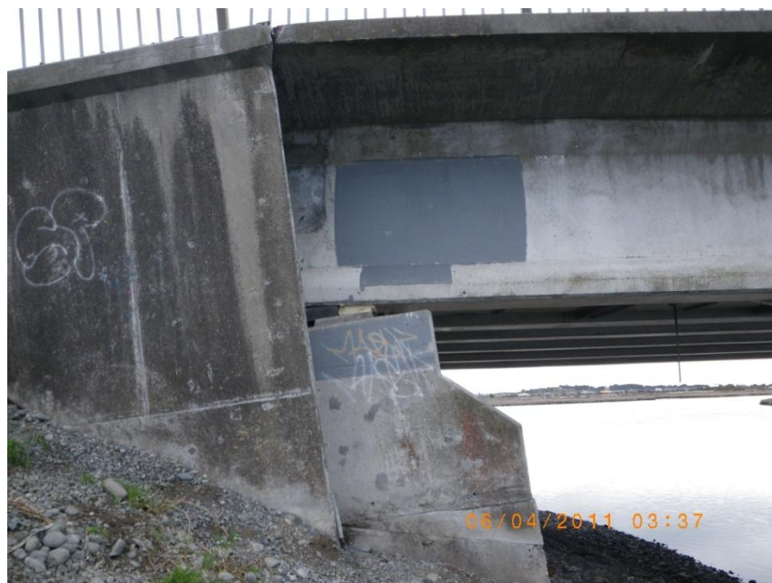
Figure 5.33. Western abutment of South Bridge Road Bridge (B8 on map of Figure 5.1) after Christchurch earthquake. Back rotation of the abutment around the deck and slump of the approach fill.
