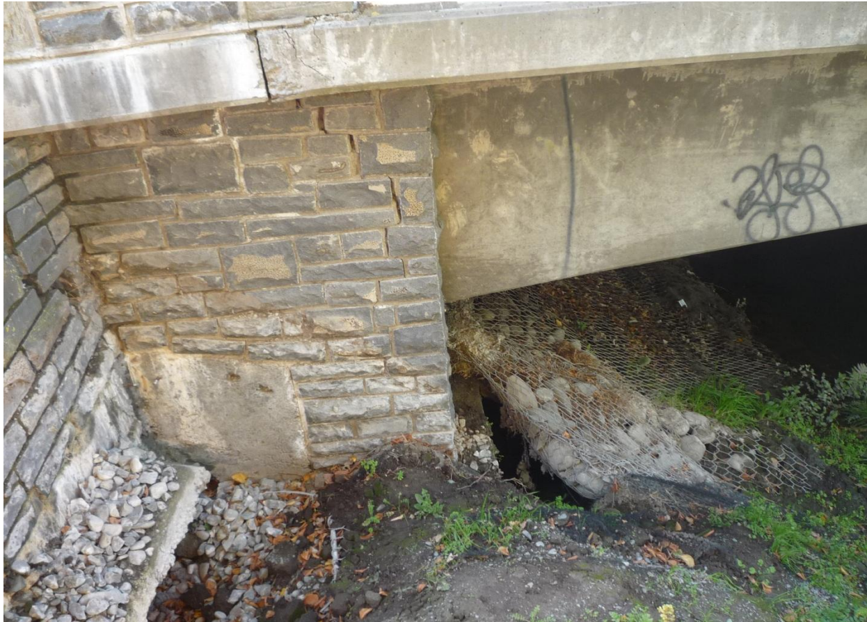
Figure 5.13. Stanmore Bridge (B2 on map of Figure 5.1). Cracks in the abutment and concrete spalling close to the joint with the deck. Gap opening between the abutment and the soil, tending to expose the foundation.
