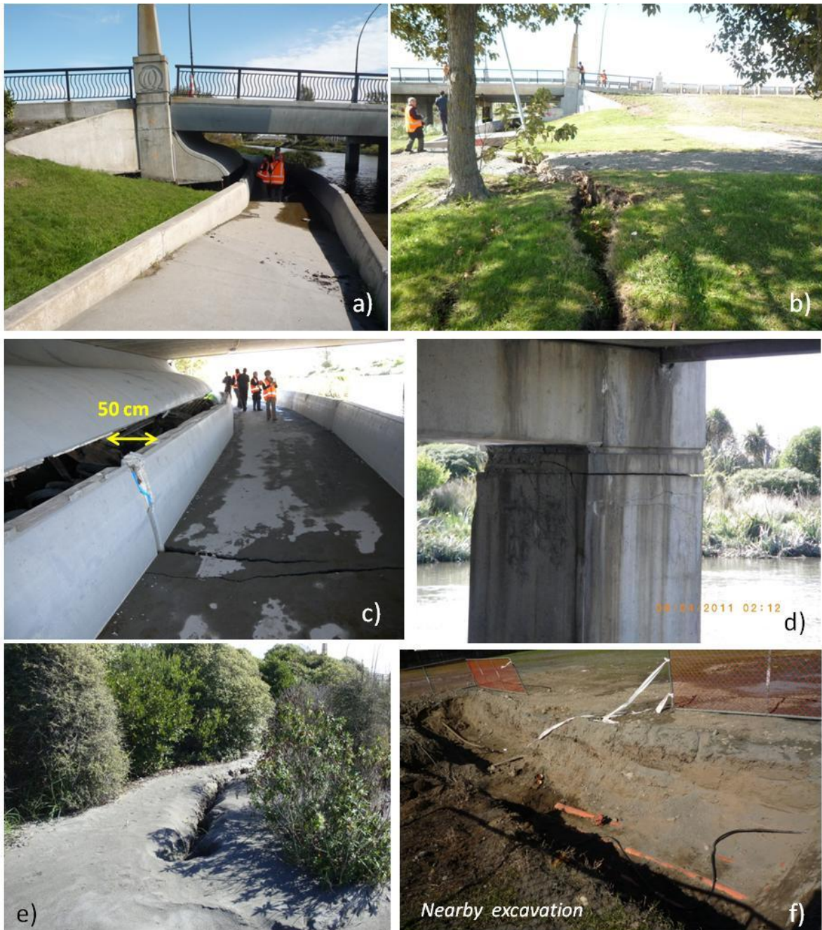
Figure 5.29. Avondale Bridge (B7 on map of Figure 5.1) after Christchurch earthquake. a) Back rotation of the abutments and slump of the approach fill, b) Large lateral spreading cracks in the ground parallel to Avon river coast extending in a great distance from the abutments indicating horizontal ground displacement more than 1, c) Riverward ground displacement in front of the abutments forms a gap of 50 cm exposing the top of the piles, d) Concrete spalling and cracks at the top of the pier-column due to intense shaking and lateral spreading, e) Significant quantity of sand ejecta close to the bridge, f) Nearby shallow excavation shows a top crust of clay containing thin beds of sand.
