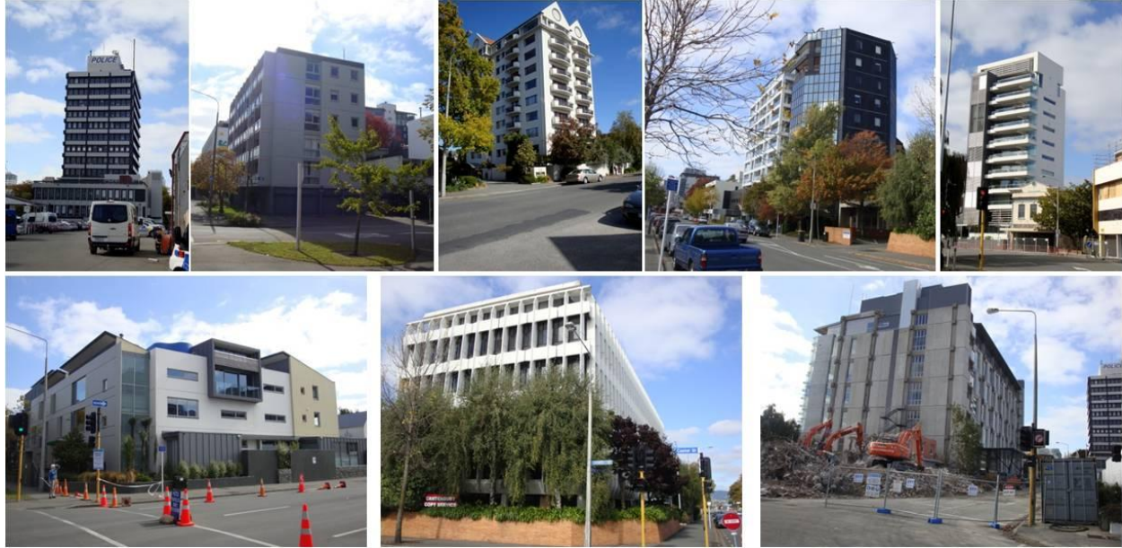
Figure 3. 56. Modern RC buildings performing satisfactorily.
