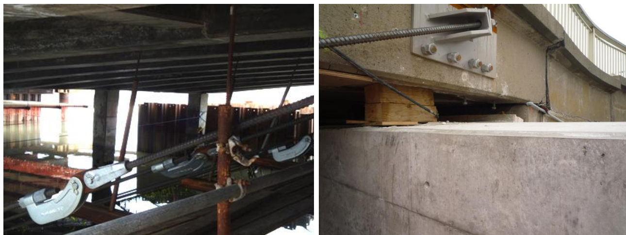
Figure 5.47. East abutment and pier of Ferrymead Bridge after Christchurch earthquake (B8 on map of Figure 5.1). The base of the piers has been tied with tendons to the edges of the deck in order to keep and restrain any inward movement (left). Timber pads have been placed between the new abutment and the deck after the earthquake (right).
