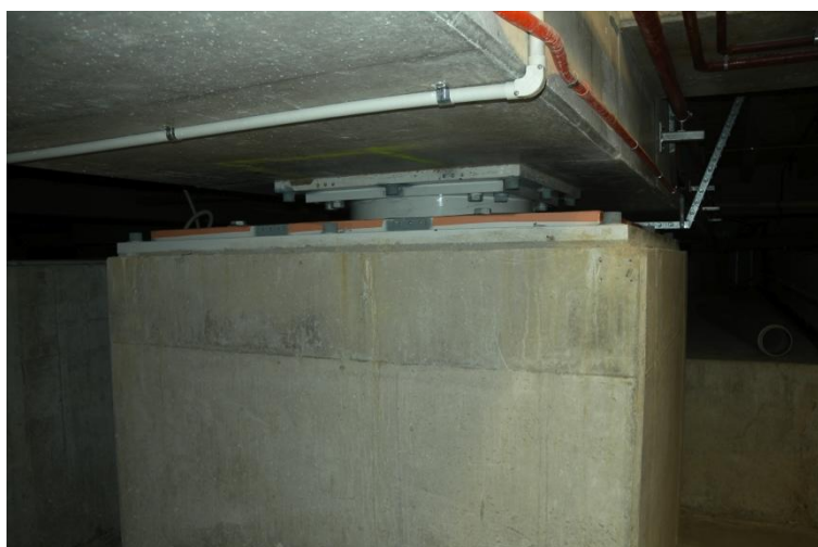
Figure 3. 43. 700mm diameter sliding bearings (double-curvature sliding mechanism).
