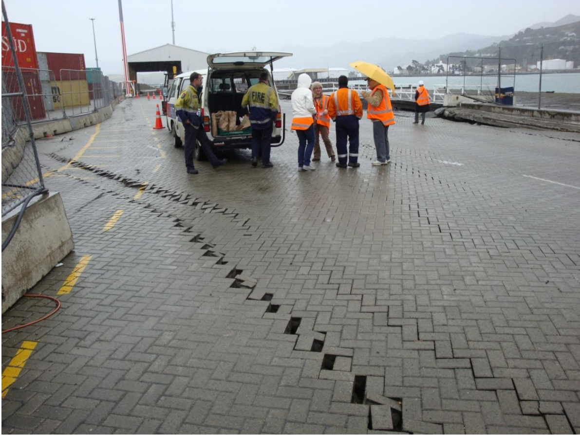
Figure 5.16. Cracks in the pavement due to lateral spreading continue to develop several meters behind the quay (site W2 pointed in the map of Figure 5.6).
