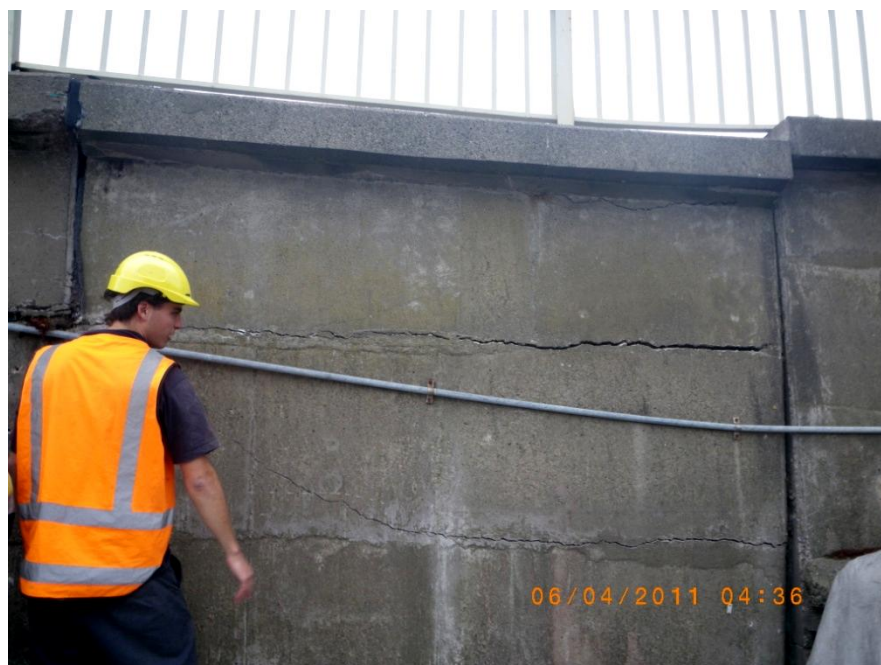
Figure 5.46. East abutment of Ferrymead Bridge after Christchurch earthquake (B8 on map of Figure 5.1). Horizontal cracks in the abutment wall have developed. The major crack is located at the height of the lower part of the deck.
