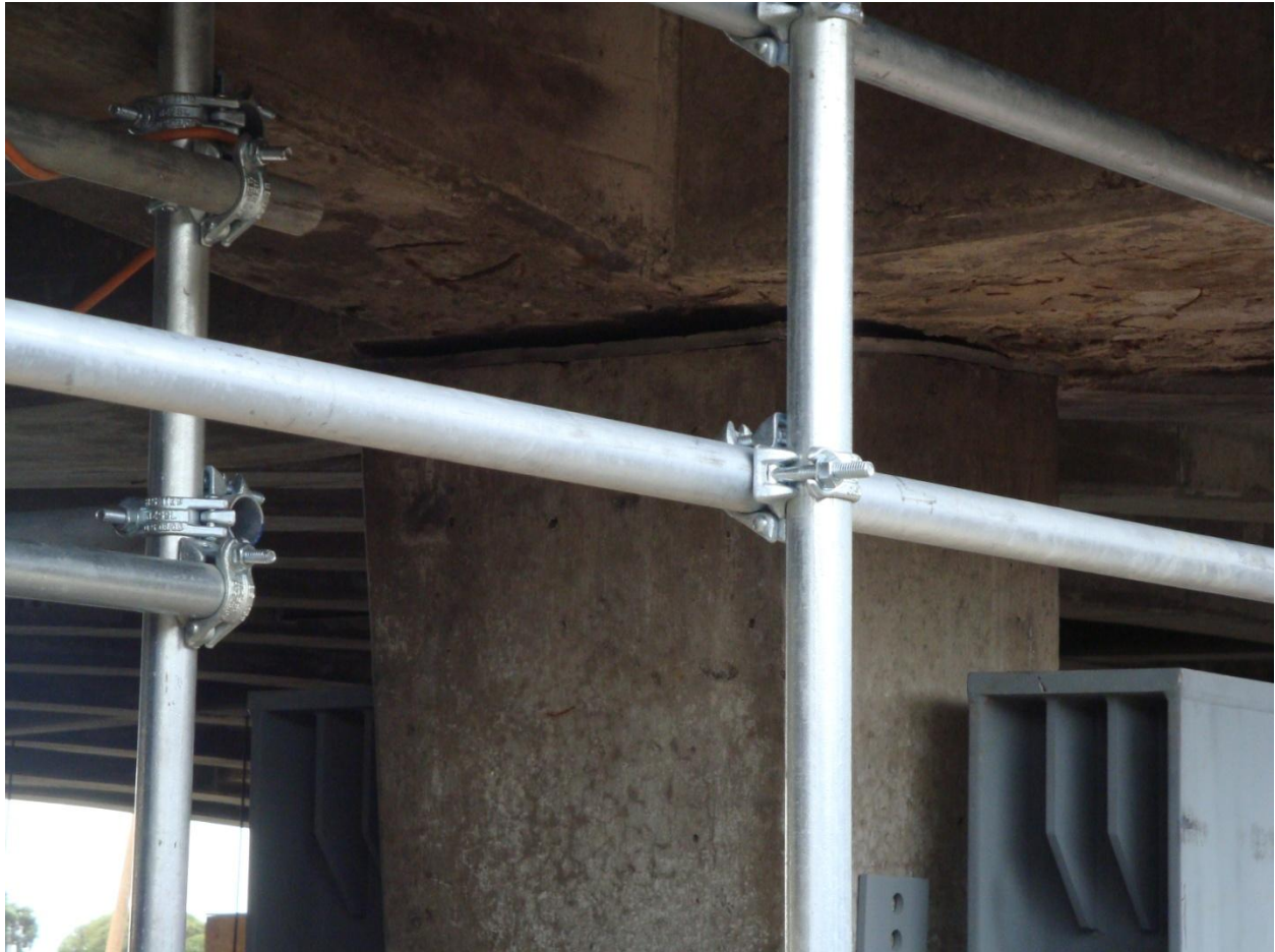
Figure 5.49. West pier of Ferrymead Bridge after Christchurch earthquake (B8 on map of Figure 5.1). The gap opening between the top of the pier and the deck was caused by the inward movement of the pier.
