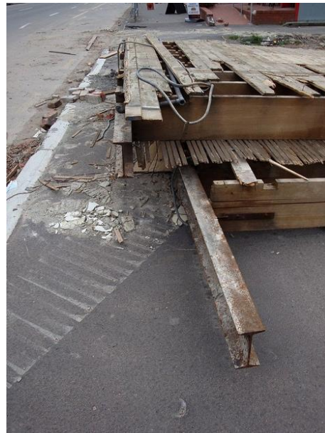
Figure 3. 5. A composite slab found at Manchester Street.
