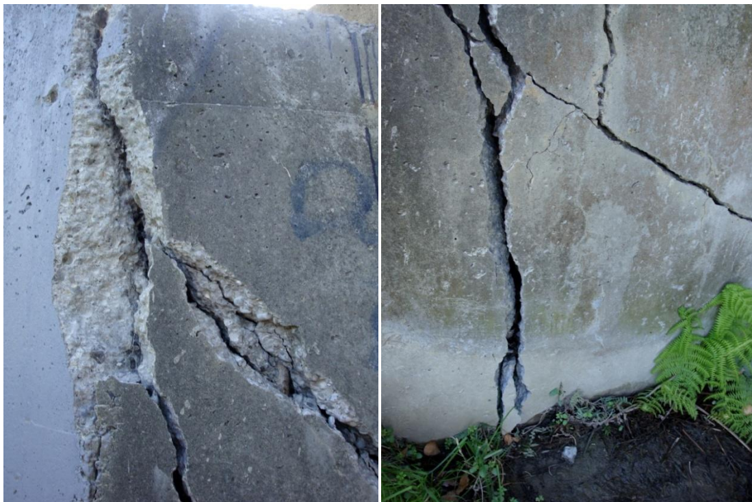
Figure 5.20. Closer look on the cracks of the western wingwall at the north of Gayhurst Bridge (B4 on map of Figure 5.1). The cracks have widened and deepened, while concrete spalling has occurred during Christchurch earthquake.
