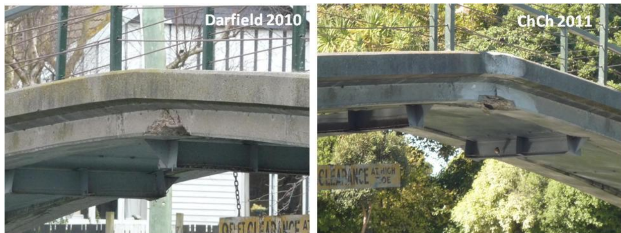
Figure 5.23. Snell Footbridge (B5 on map of Figure 5.1) after Christchurch earthquake. Comparison of damage between Darfield and Christchurch shaking events. The cracks have widened and extended at the mid-point. Source: NHP- Bridge Research Group.
