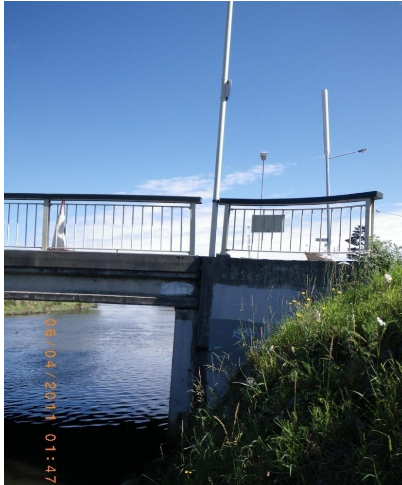
Figure 5.28. Northern abutment of Avondale Bridge (B6 on map of Figure 5.1) after Christchurch earthquake. Moderate back rotation (4 degrees) with only slight settlement of the backfill.
