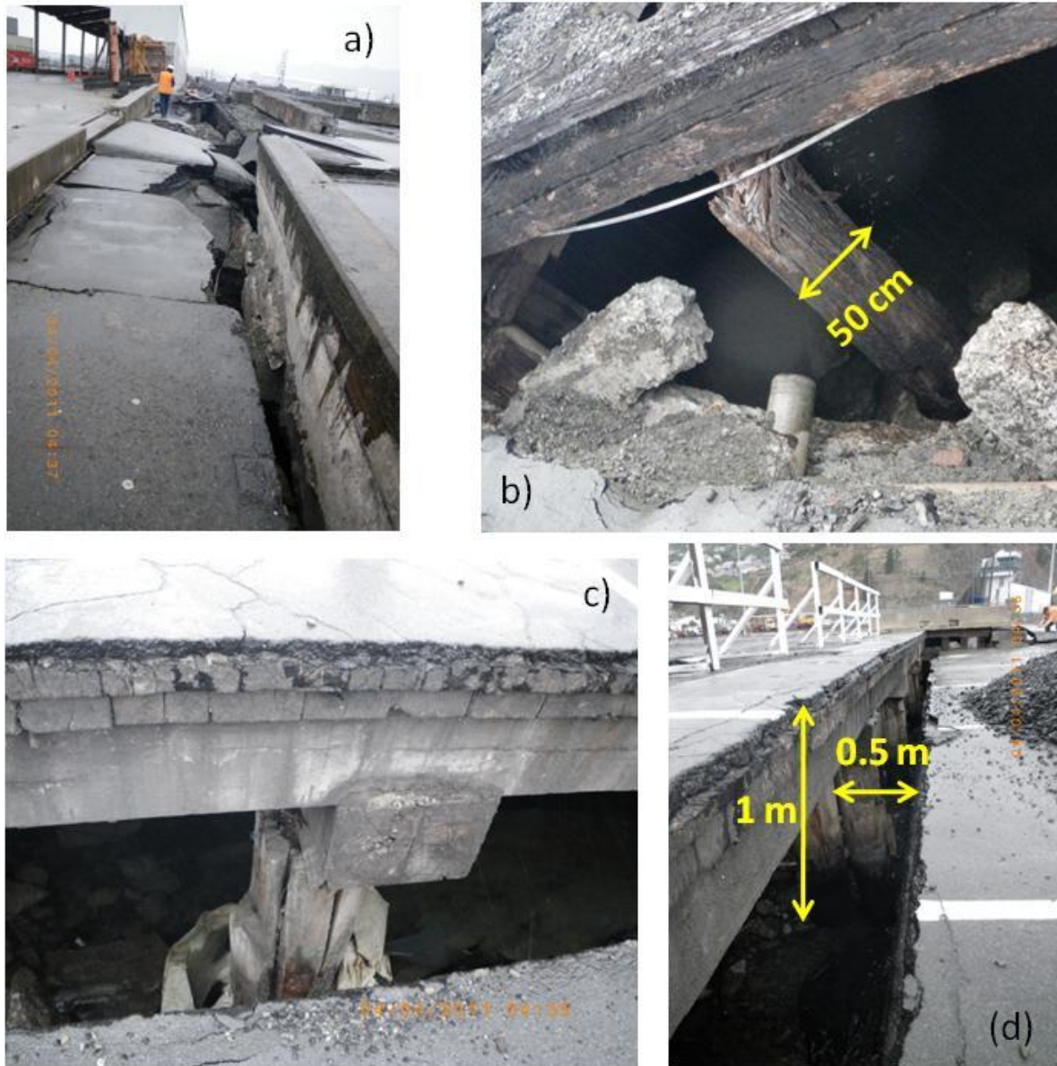
Figure 5.17. Damage of the container terminal quay (site W2 pointed in the map of Figure 5.6): a) Crack opening and distortion of the asphalt connecting the terminal with the wharves, b) Plastic hinging at the top of a timber pile of 50 cm diameter, c) Relative movement of the deck to the pile, d) Separation of the wharf to the backfill due to 1 m settlement of the backfill and outward movement of the wharf up to 50 cm.
