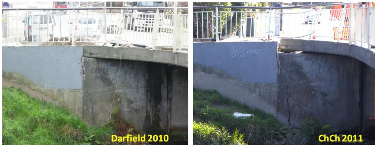
Figure 5.19. Western side of the northern abutment of Gayhurst Bridge (B4 on map of Figure 5.1). Comparison of damage between Darfield and Christchurch shaking events. The cracks have widened and extended, while the differential lateral riverward displacement of the abutment and wingwalls relative to the deck has increased after Christchurch earthquake Source: NHP-Bridge Research Group.
