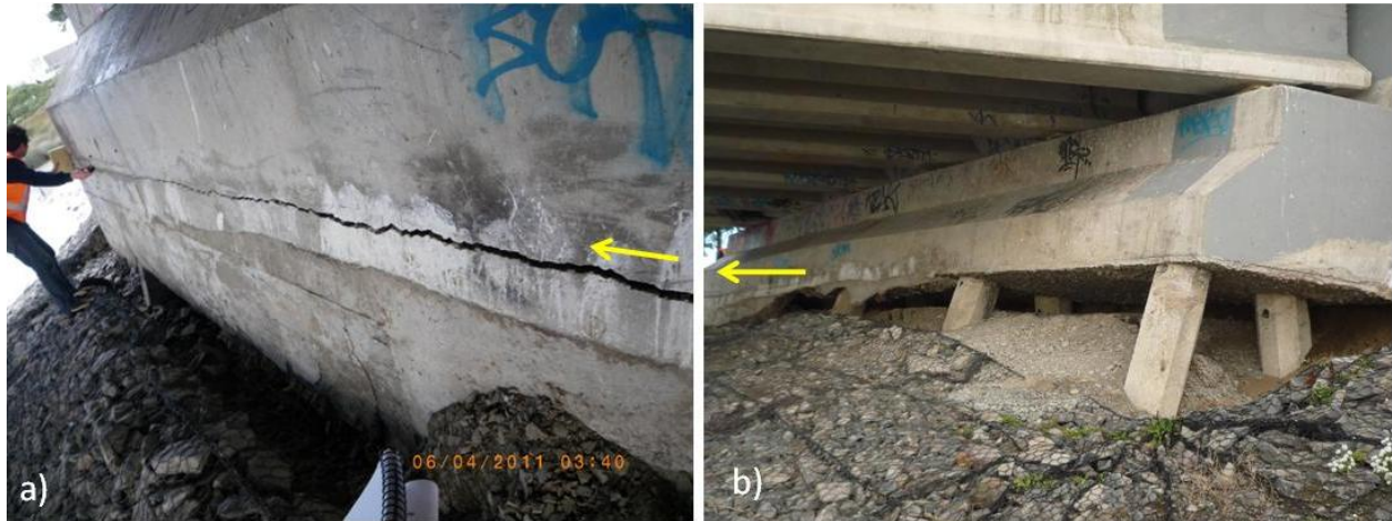
Figure 5.34. Western abutment of South Bridge Road Bridge (B8 on map of Figure 5.1) after Christchurch earthquake. a) Large tension horizontal crack at the base of the abutment, b) The gabion mat used for erosion protection in front of the abutment has laterally and vertically moved so that a great part of the pile heads has been exposed.
