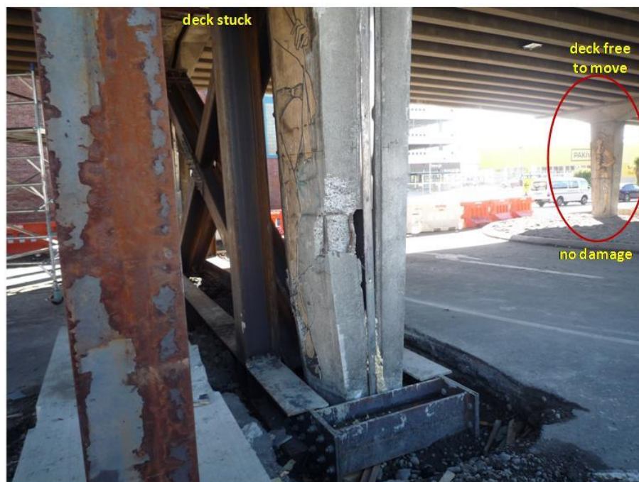
Figure 5.52. Failure of the pier due to shear and then buckling of the rebar under axial loads.
