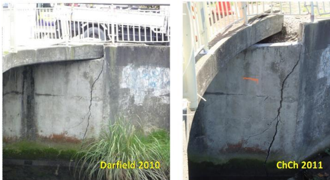
Figure 5.21 Eastern side of the northern abutment of Gayhurst Bridge (B4 on map of Figure 5.1). Comparison of damage between Darfield and Christchurch shaking events. The cracks have widened and the differential lateral riverward displacement of the abutment and wingwalls relative to the deck has increased after Christchurch earthquake. SOURCE.
