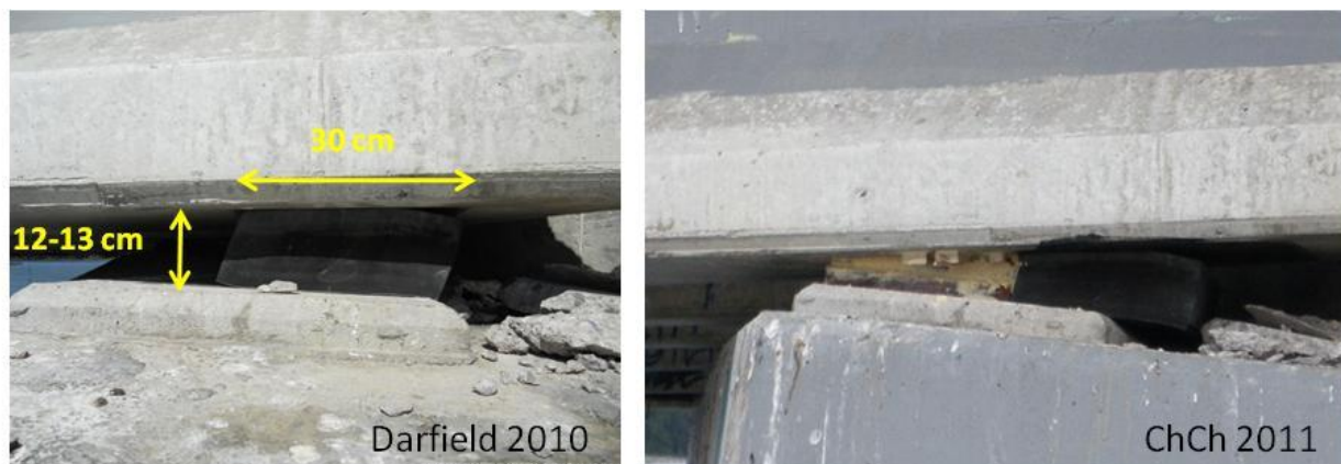
Figure 5.38. Western abutment of South Bridge Road Bridge (B8 on map of Figure 5.1). Differences between Darfield and Christchurch shaking events. The rubber bearing pad had sheared and slid laterally in Darfield earthquake. After Christchurch earthquake the rubber pad has deformed and displaced even more. The timber pad, used as a stop probably has been placed after Darfield earthquake, because it seems to have sustained certain deformation. Source: NHP- Bridge Research Group..
