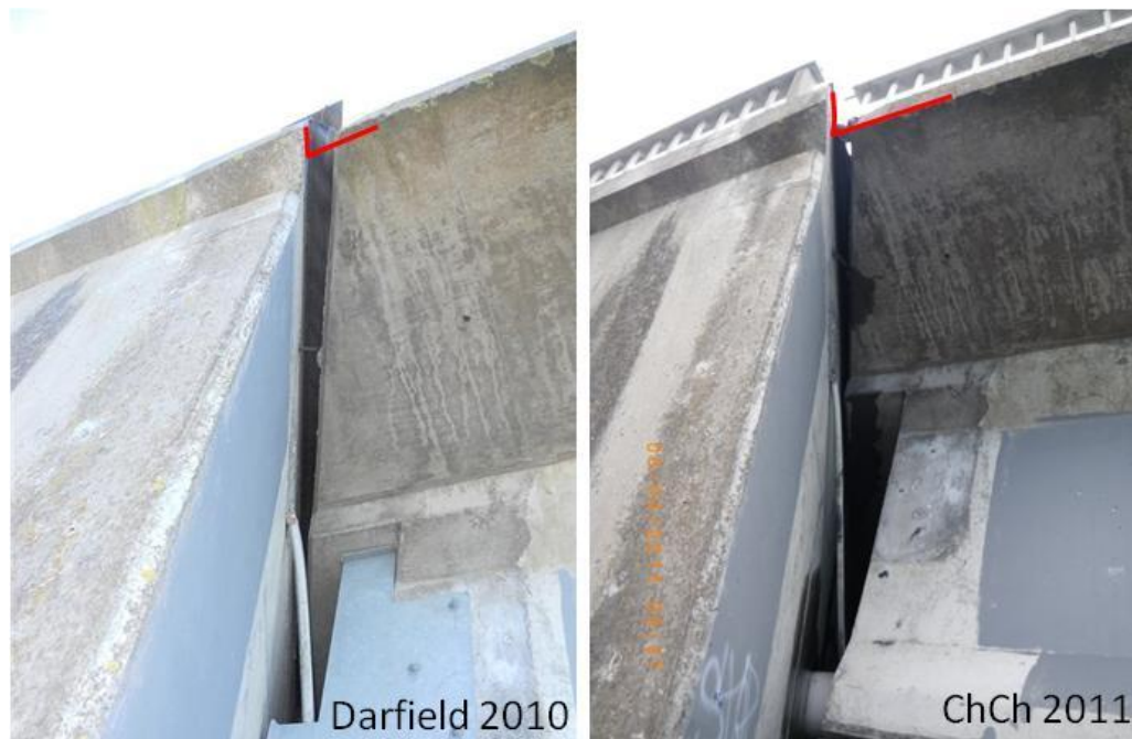
Figure 5.40. Western abutment of South Bridge Road Bridge (B8 on map of Figure 5.1). Slight differences between Darfield and Christchurch shaking events in terms of differential displacement of the abutment relative to the deck in the skew line direction. Source: NHP-Bridge Research Group.
