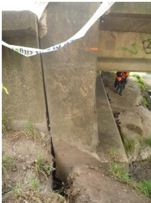
Figure 5.5. Fitzgerald Bridge (B1 on map of Figure 5.1). Performance of northern abutment after ChCh earthquake. Rotation of abutment is evident due to lateral spreading. The backfill has differentially subsided relative to the abutment.
