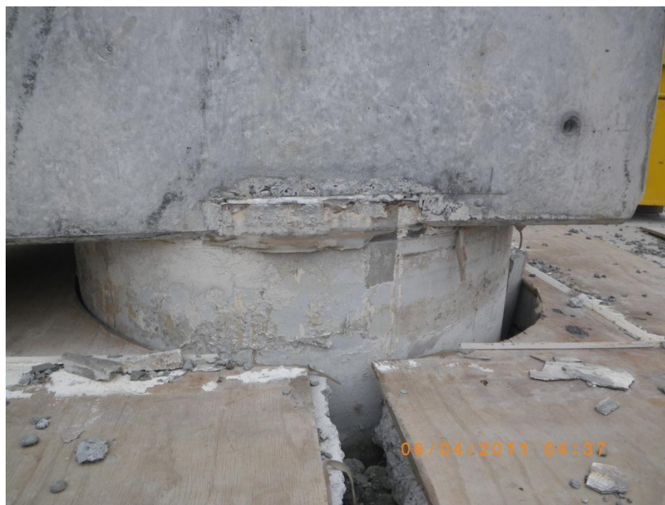
Figure 5.48. New east abutment of Ferrymead Bridge after Christchurch earthquake (B8 on map of Figure 5.1). The abutment have moved towards the center of the bridge. The gap opening at the back side of the pile is a result of this movement.
