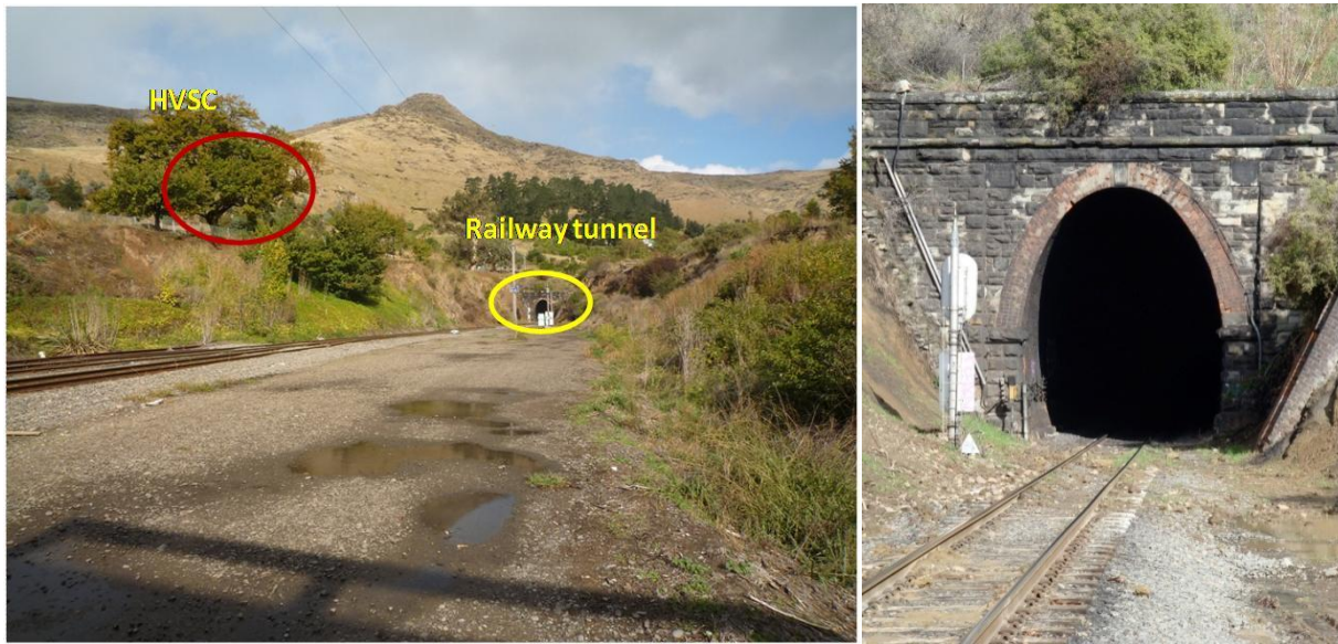
Figure 2.48. The excavation adjacent to HVSC station, leading to railway tunnel. The remnants of rain water show that it cannot be easily absorbed by the soil which is indicative of clayey soil with low permeability(left). The entrance to the railway tunnel showing, no damage (right).
