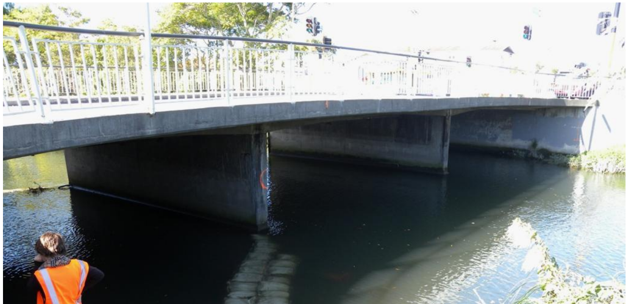
Figure 5.15. Gayhurst Bridge (B4 on map of Figure 5.1) after Christchurch earthquake. The southern abutment appears practically undamaged on the right side of the photo.
