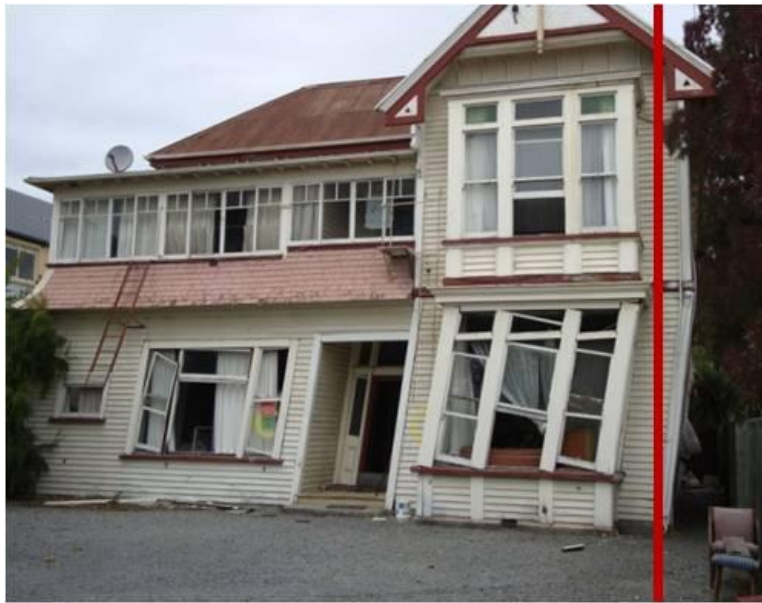
Figure 3. 6. Collapsed wooden residence at Gloucester St.
