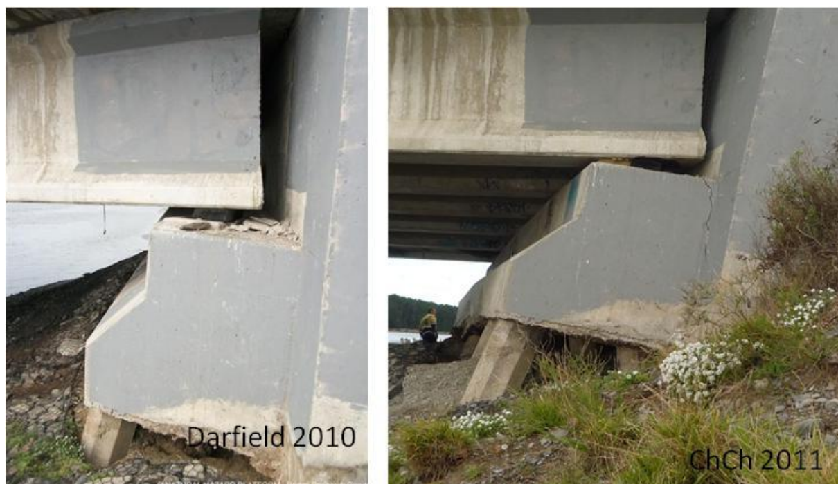
Figure 5.39. Western abutment of South Bridge Road Bridge (B8 on map of Figure 5.1). Differences between Darfield and Christchurch shaking events. After Christchurch earthquake the piles have been more exposed due to greater lateral spreading of the soil and some cracks have been developed in the abutment. Source: NHP- Bridge Research Group.
