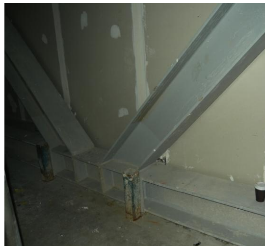
Figure 3. 40. Eccentrically placed steel bracing in the superstructure of the Women's Hospital.
