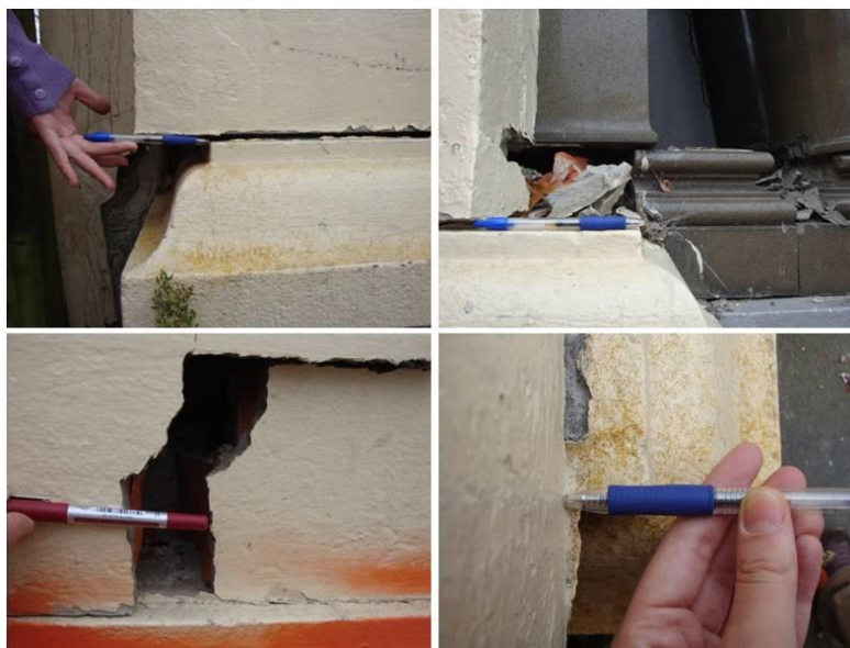
Figure 3. 12. Lateral displacement of columns in the EW direction.
