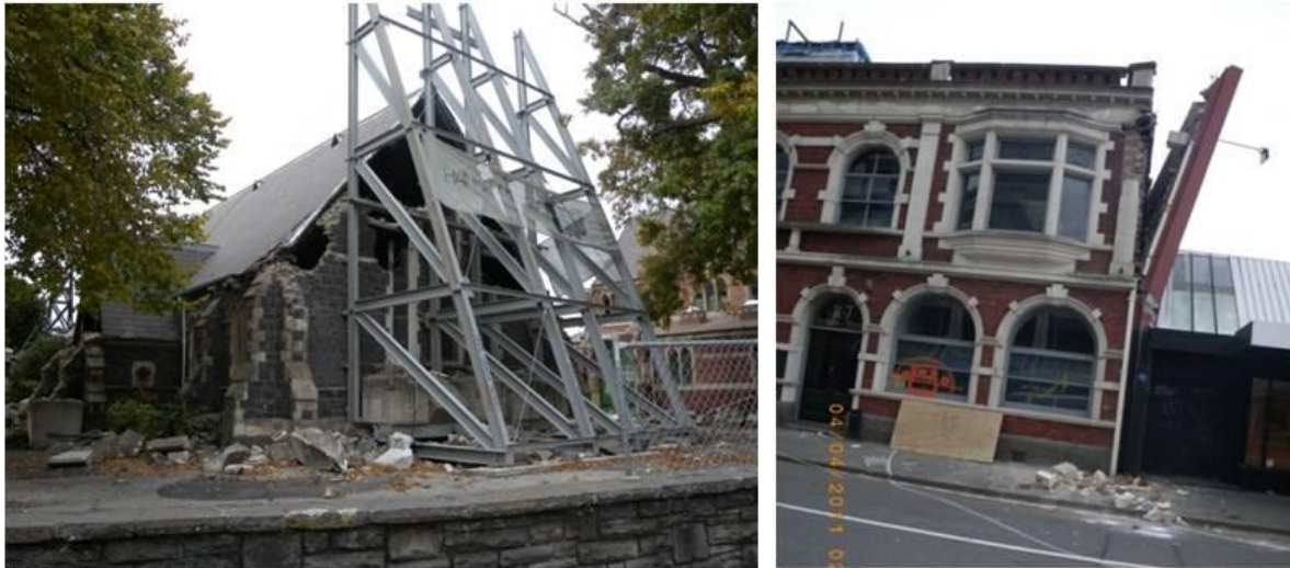
Figure 3. 16. Out-of-plane failures around Hereford Street.
