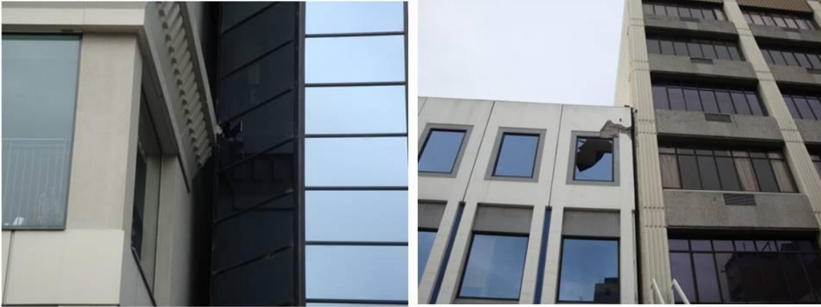
Figure 3. 22. Observed pounding effect in CBD.
