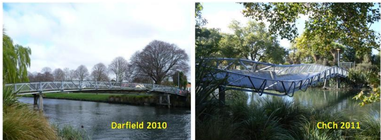
Figure 5.14. Medway Pedestrian Bridge (B3 on map of Figure 5.1). Comparison of bridge damage between Darfield and Christchurch earthquakes. Source: NHP- Bridge Research Group.
