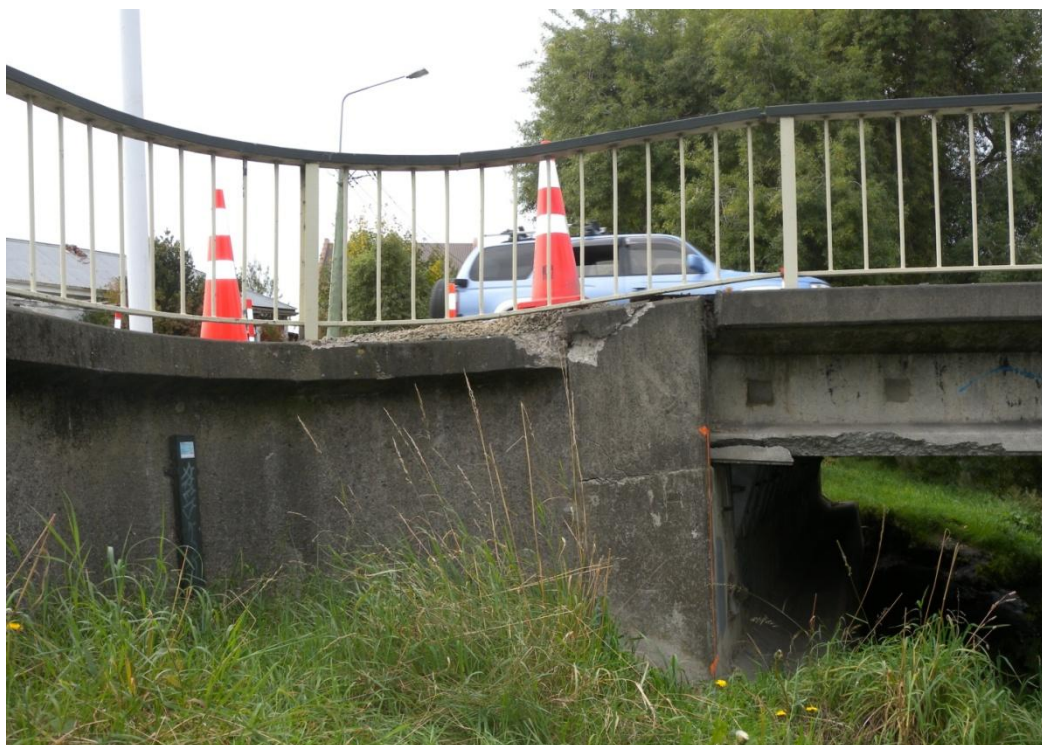
Figure 5.7. Fitzgerald Bridge (B1 on map of Figure 5.1). Performance of northern abutment of the twin bridge after ChCh earthquake. Rotation of abutment and slump of the backfill took place. Concrete spalling of the deck developed close to the abutment-seat.
